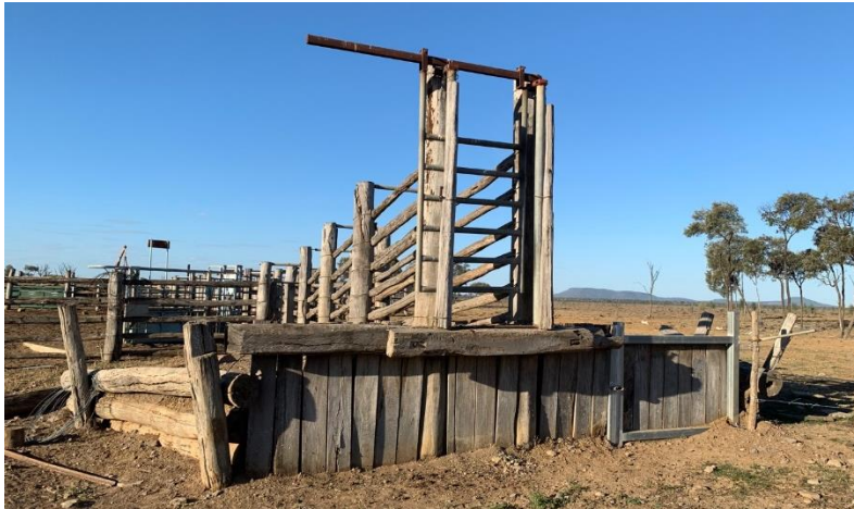
Figure 85. View north of the cattle loading ramp at WS27. The ramp is of timber and earthen construction, reinforced with metal elements.
