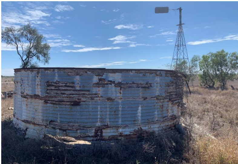
Figure 55. View north of WS14, being the remains of a corrugated iron water tank.
