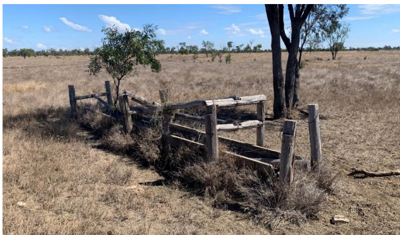
Figure 46. View north-west of WS11, a concrete water trough with a timber post-and-rail frame.
