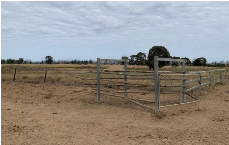
Figure 20. View towards WS02 – cattle yards constructed using a combination of metal post-and-rail and timber posts strung with wire. Note the cattle sorting gate in the centre of frame, constructed using a combination of metal uprights and horizontal rails, and narrow timber rails.
