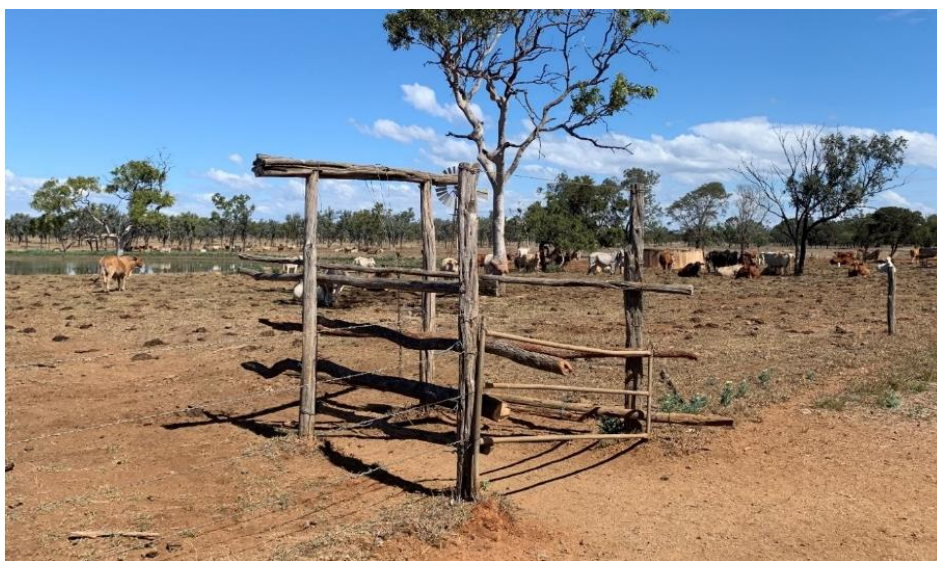
Figure 62. View south-west of WS16, showing the main cattle sorting gate constructed using a combination of timber posts and rails, metal wire, and a metal gate.
