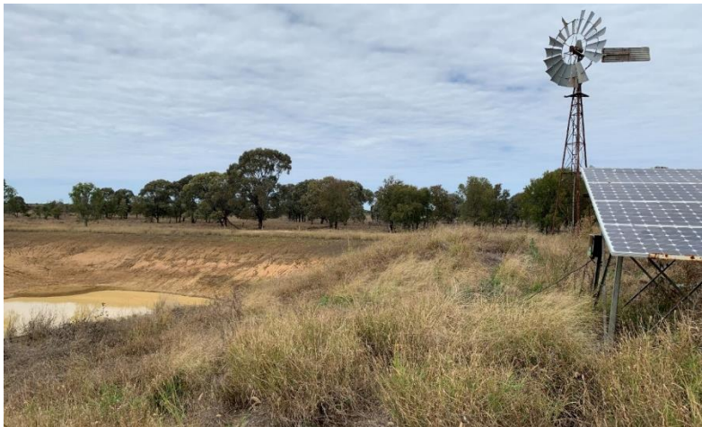
Figure 23. View facing south of WS03, showing one of the dams and the associated windmill. Note the modern addition of solar panels providing power to the windmill.
