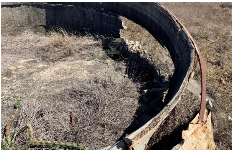
Figure 57. View west showing the remains of the concrete slab foundations of the water tank.
