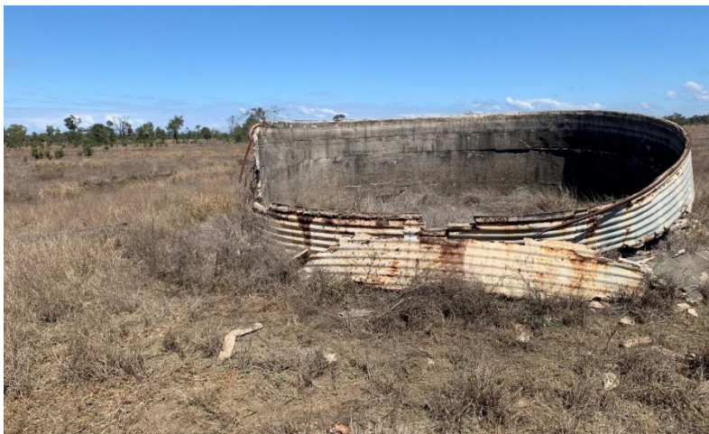
Figure 56. View south of WS14 showing the concrete lining and corrugated iron sheeting. Note the tank is in a state of partial collapse and the corrugated iron sheeting is corroded.
