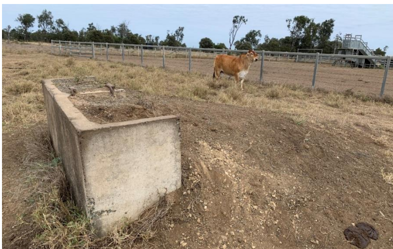
Figure 28. View south towards WS04 showing the concrete block structure located adjacent to the eastern boundary of the cattle yards. This concrete block is held together by metal rods and packed with earth, and may have been used as a modified cattle-loading ramp.
