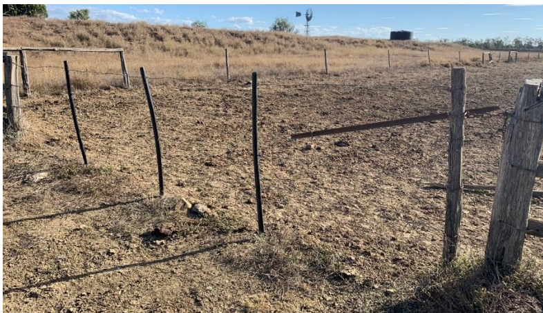
Figure 81. View facing south-west showing a section of the WS25 cattle yard fencing, where the timber posts have been replaced with modern PVC piping and strung with wire.
