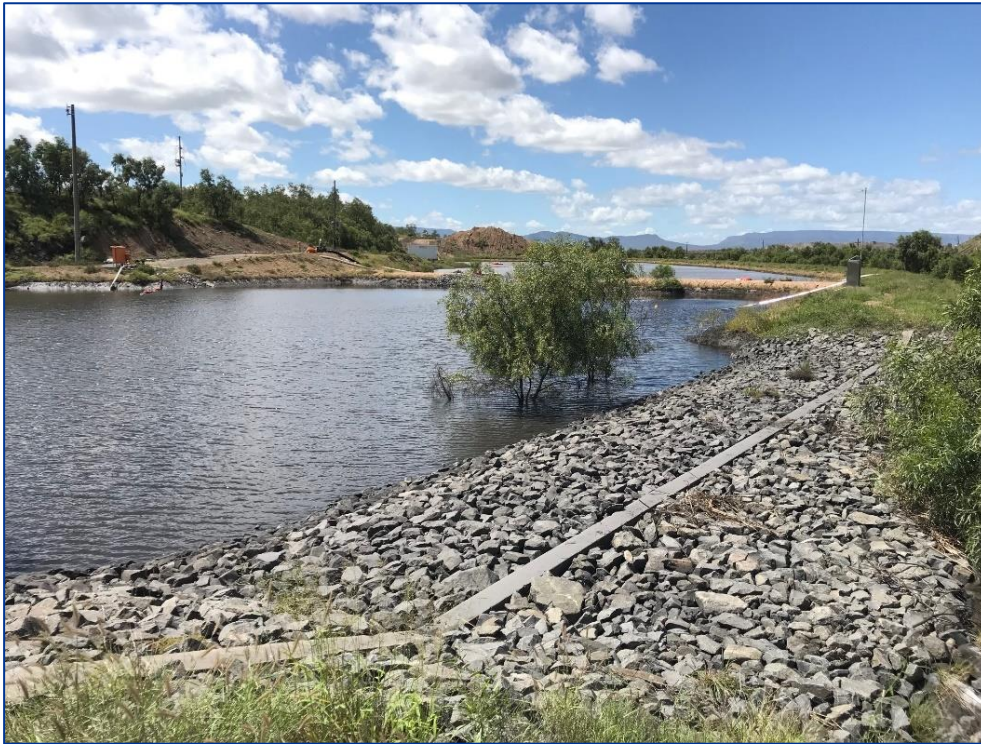
Plate 3-7A – Example of Riprap-lined Spillway
