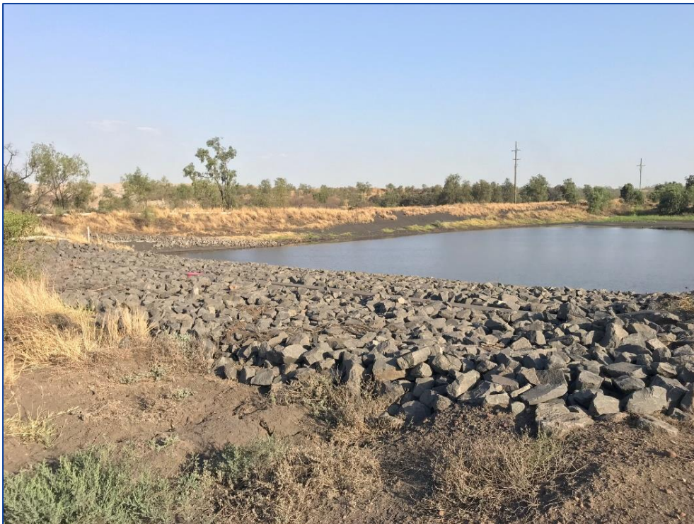
Plate 3-7B – Example of Riprap-lined Dam Bank
