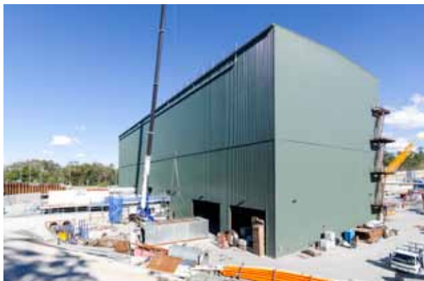
Ventilated acoustic shed, Legacy Way
