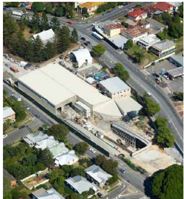
Airport Link–Northern Busway worksite
