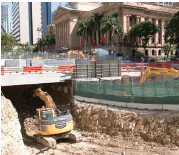
Construction, King George Square Busway
