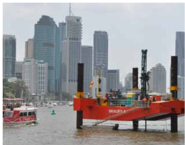
Geotechnical drilling, Brisbane River
