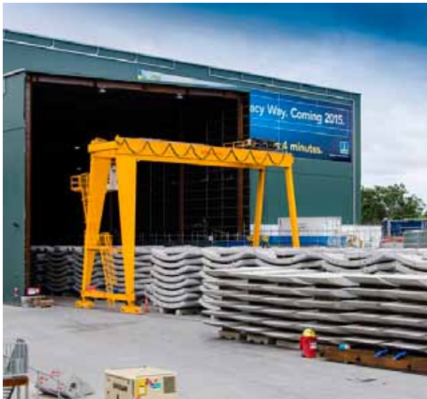
Precast concrete segments, Legacy Way Image courtesy of Rix Ryan Photography
