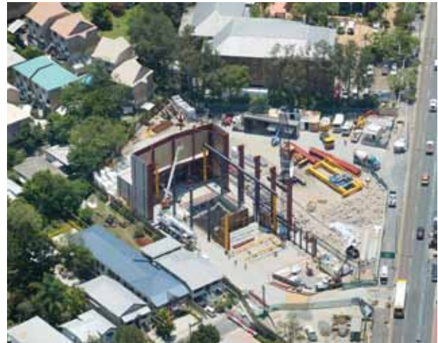
Construction of Kangaroo Point workshed, CLEM7 Photo courtesy of Brisbane City Council
