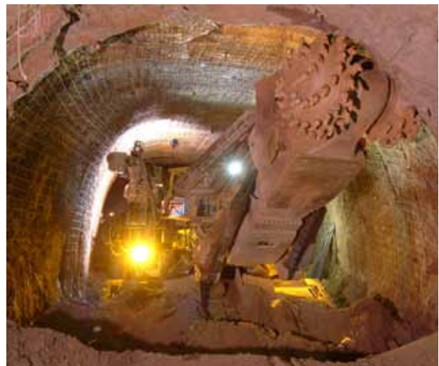
Roadheader construction
