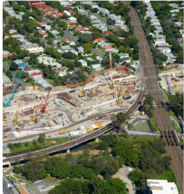
Kalinga Park worksite, Airport Link
