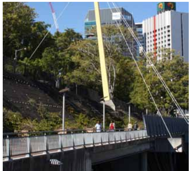
Albert Street pedestrian link, Roma Street Parkland
