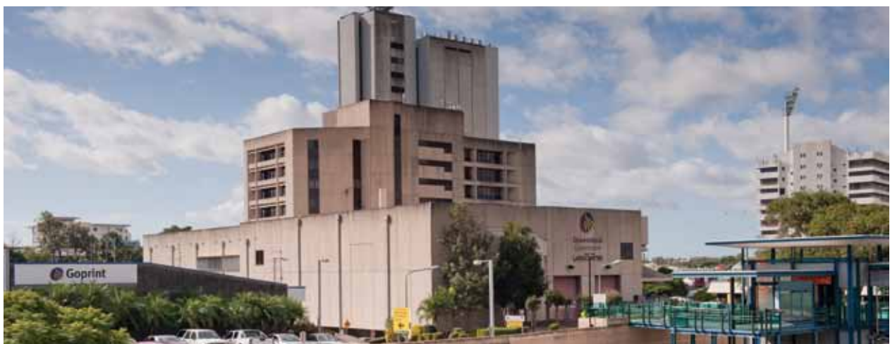
Goprint Building and Land Centre, Woolloongabba
