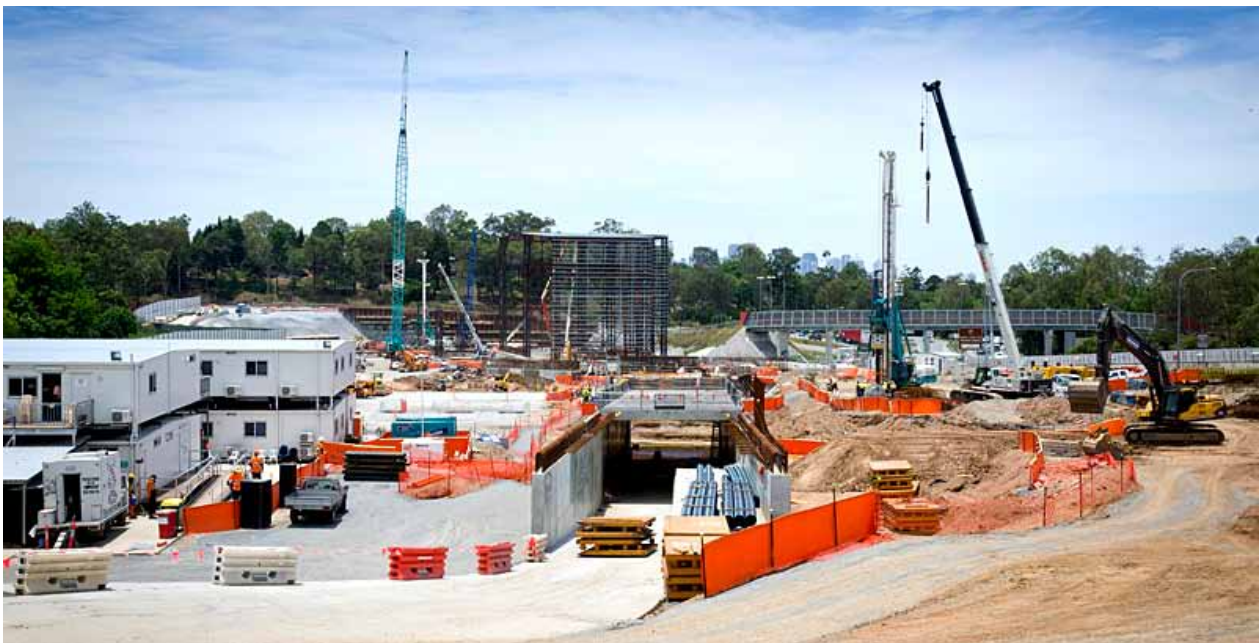
Construction worksite, Legacy Way Image courtesy of Rix Ryan Photography
