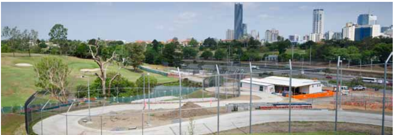
Worksite, Legacy Way (Image courtesy of Rix Ryan Photography)
