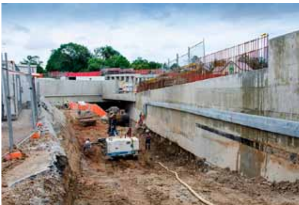
Portal construction, Legacy Way Image courtesy of Rix Ryan Photography
