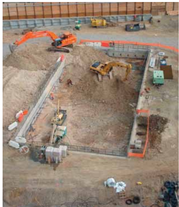
Excavation works – tunnel shaft Photo courtesy of Brisbane City Council
