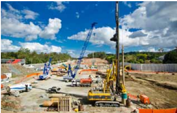
Piling, Legacy Way Tunnel
