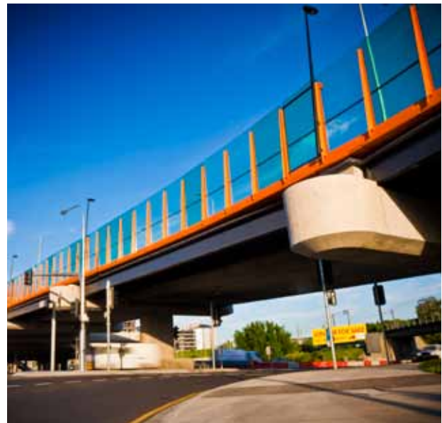
Busway bridge – Eastern Busway, Woolloongabba
