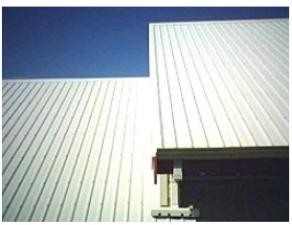
White Roof. The most cost effective energy (and greenhouse) solution for new homes in Townsville is to ensure that the roofs are white or as light in colour as possible. White has a high albedo, which is the reflectance of solar energy. The more solar energy that is reflected, the less is absorbed as heat into the building. Hot houses are energy hungry houses.
