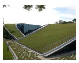
Green Roofs. Roofs should either be white or green or covered in solar panels (if you are not going to use the sunshine, send it back). Green roofs are roofs that have special substrates that permit the arowth of vegetation. Green roofs are lasting, attractive and cool. With the right selection of plants, the roof functions like an evaporative air conditioner.
