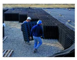
Storm water storage. Build multi-mega-litre storm-water storage infrastructure throughout the site. This will not only reduce total amount of fill required, but will also reduce the development's impost on the water supply infrastructure. The system shown here, can be used under roads and park lands.
