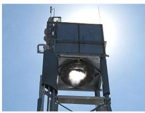
Centralized solar power **station.** Produce all energy requirements from on-site power stations. Shown here is the receiver of the Lloyd Energy solar heliostat. This graphite to store heat allows the steam turbines to run after the sun has gone down. A 10 MW power station using this Australian technology is built in North being Queensland.
