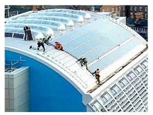
Building Integrated Photo-voltaics. Modern solar power systems actually form part of the building envelope. These systems not only provide power but also offset some of the costs of the building materials. Shown here is a climate sensitive building using BIPV in the UK. The Cruise Ship Terminal should be designed for the Townsville Climate using extensive BIPV.
