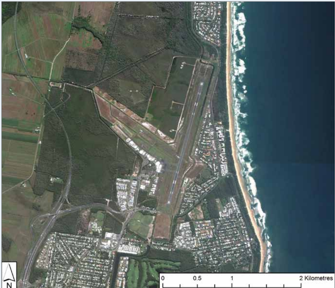
Figure 16.4d: Aerial imagery of the SCA Project site (Google Earth, 2013). Residences directly to the east of the north-south runway are most likely to be impacted during the construction phase of the project by dust emissions
