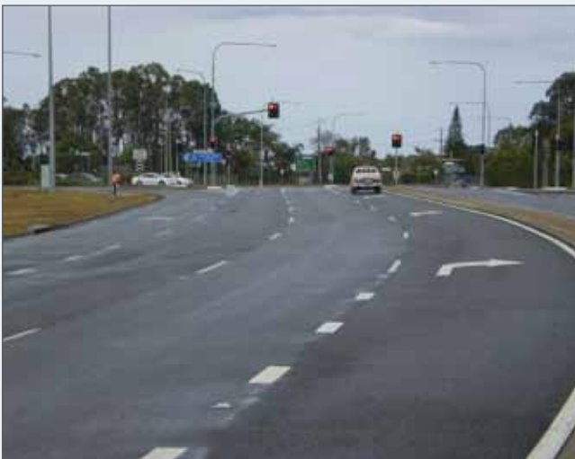
Bottom left: Image looking east along David Low Way towards the David Low Way/Airport Drive intersection
