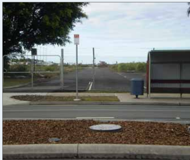
Bottom right: Image looking north towards the existing bus stop along David Low Way, with Friendship Avenue (closed) shown in the background
