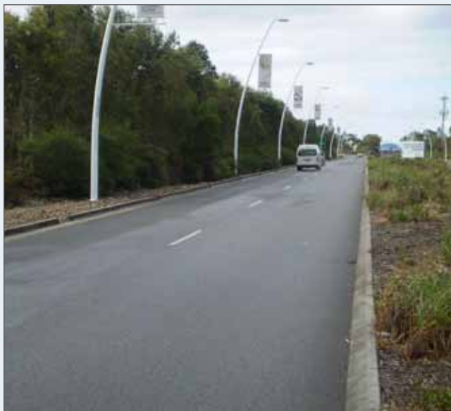
Top right: Image looking north along Airport Drive showing approach lanes to the airport
