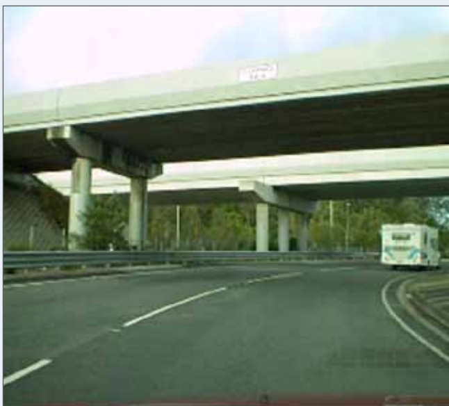
Bottom left: Image looking east at the Sunshine Motorway/David Low Way intersection showing the roundabout circulating lanes and Sunshine Motorway overpass
