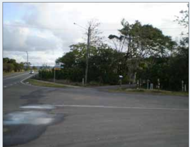
Bottom right: Image looking west along David Low Way from the David Low Way/Finland Road intersection showing the limited sight distance and property access next to the intersection
