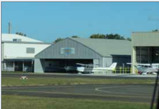
Figure 12.2n: Sunshine Coast Aero Club – airside view
