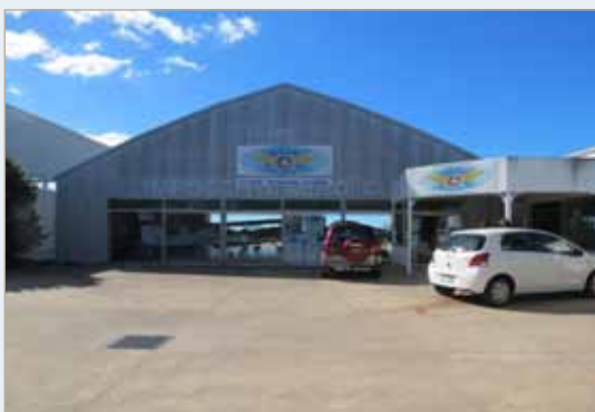
Figure 12.2p: Sunshine Coast Aero Club - hangar and club rooms
