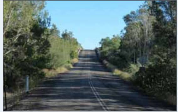
Figure 12.2w: Bitumen section of road – Bridge over the Sunshine Motorway
