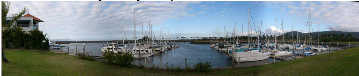
Figure 5: Laguna Quays Marina Panoramic View
