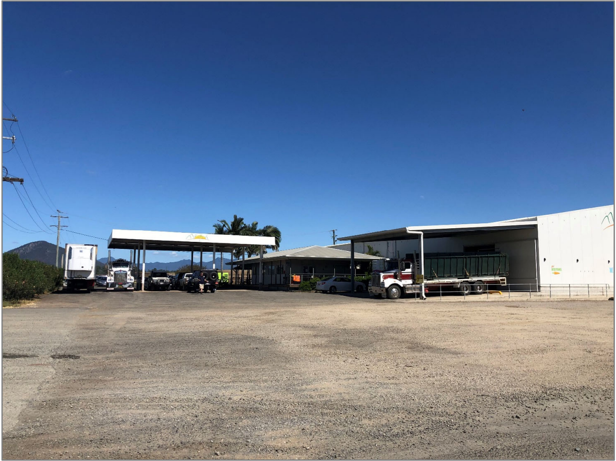
Figure 7 View of existing structures on site looking south
