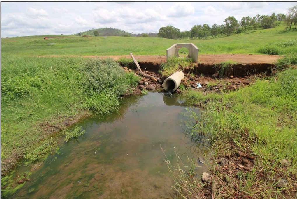
Site 4 – Small pool below culvert crossing contained fish. Culvert acting as barrier to fish passage.
