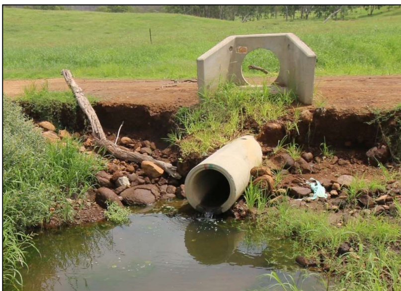
Figure 5. The waterway crossing that is acting as a barrier to fish passage.
