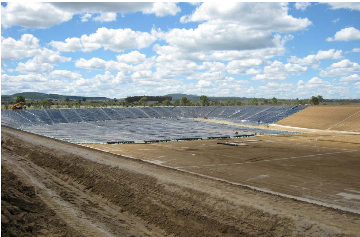
Plate 4-5 Laying liner during construction of water storage structure
