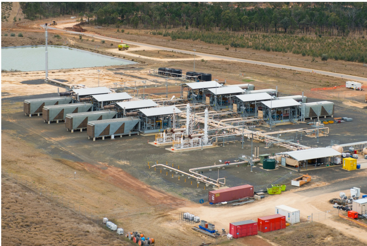
Plate 4-9 Existing nodal gas compression and treatment facility at Fairview gas field
