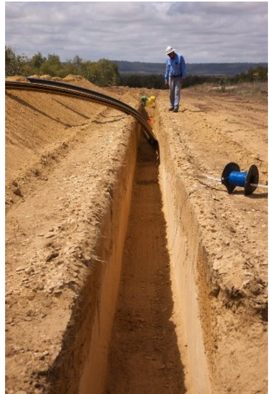
Plate 4-2 Laying transmission pipeline in Fairview
