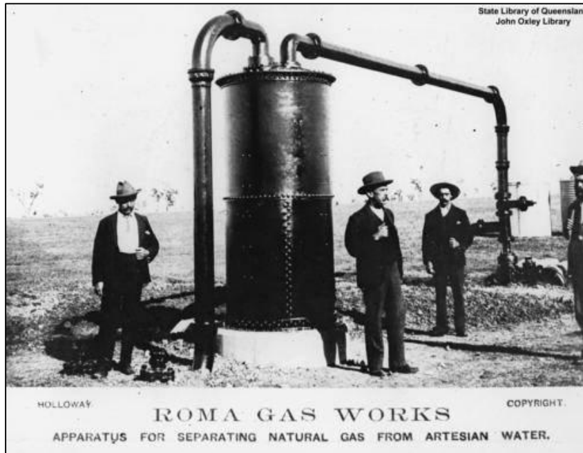
Figure 12: Apparatus for separating natural gas from artesian water at Romas Gas Works, Qld, c. 1906 (JOL Image number: 39114)
