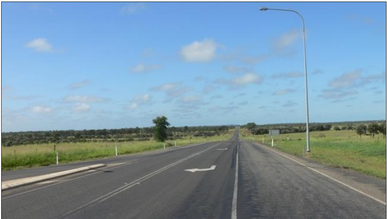
Figure 7-7 Goonyella Road/Red Hill Road Intersection: Southern Goonyella Road Approach - Looking South
