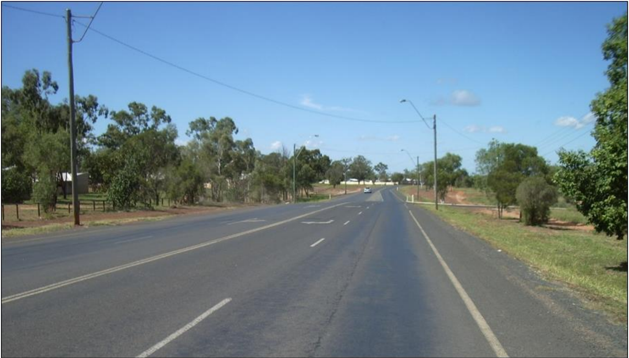
Figure 7-11 Goonyella Road/Curtin Street Intersection: Southern Goonyella Road Approach - Looking South
