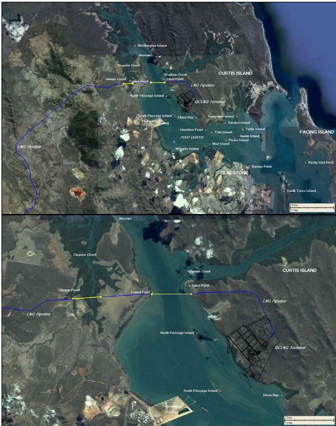
Figure 2: Large scale view (top) and zoomed in view (bottom) of the proposed QCLNG facility and layout of the natural gas pipeline (denoted in blue) within Port Curtiss. (Note: yellow lines represent the marine based sections examined as part of the sediment dispersion modelling assessment).
