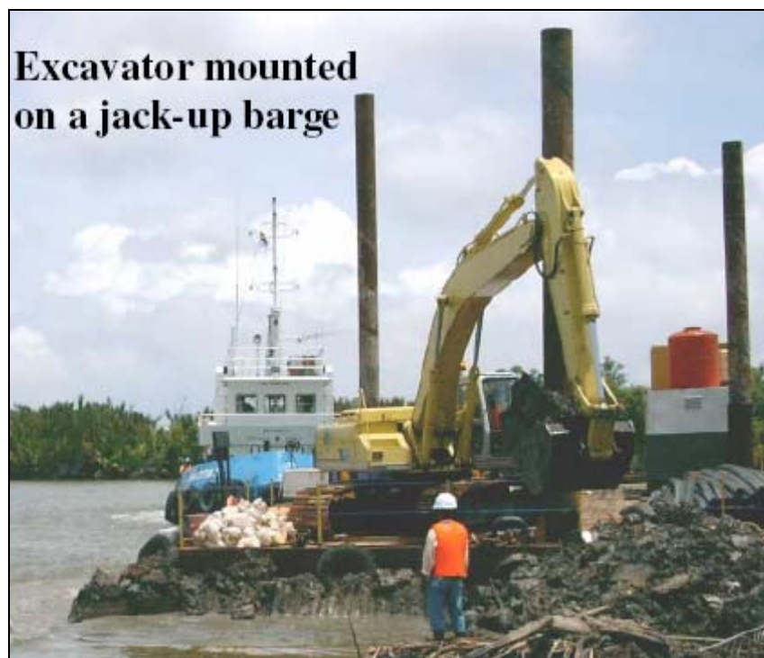
Figure 9: Photograph of a BHD on a barge for dredging of marine sediments (Source: Xodus Group Pty. Ltd., 2009).
