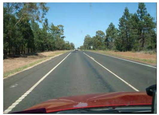
Figure 2.8 Warrego Highway 18D (Miles-Roma) – sealed shoulders (state controlled)
