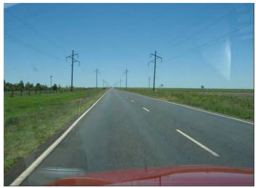
Figure 2.2 Warrego Highway east of Dalby – unsealed shoulders (state controlled)
