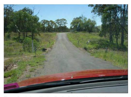
Figure 2.5 Jackson–Wandoan Road – single lane bitumen floodway – no line marking (state controlled)
