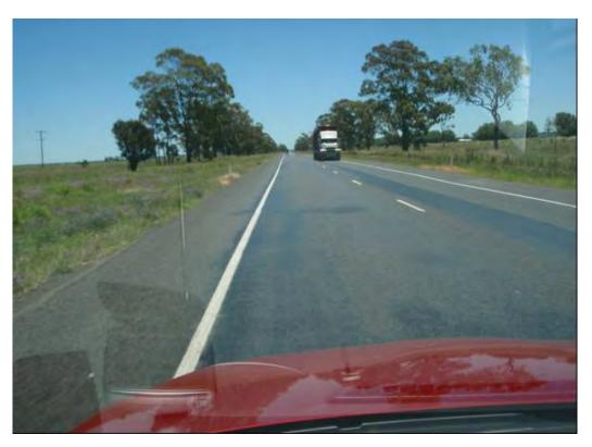
Figure 2.1 Warrego Highway west of Oakey – 2m wide sealed shoulders (state controlled)
