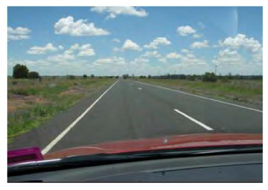
Figure 2.3 Leichhardt Highway 26B (Taroom-Miles) – sealed shoulders (state controlled)
