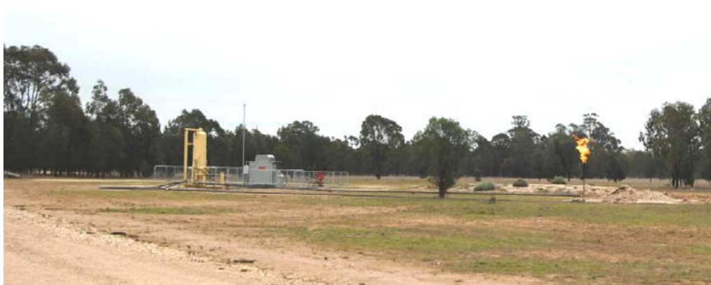
Figure 3.15.4 Typical Gas Separator and Flare
