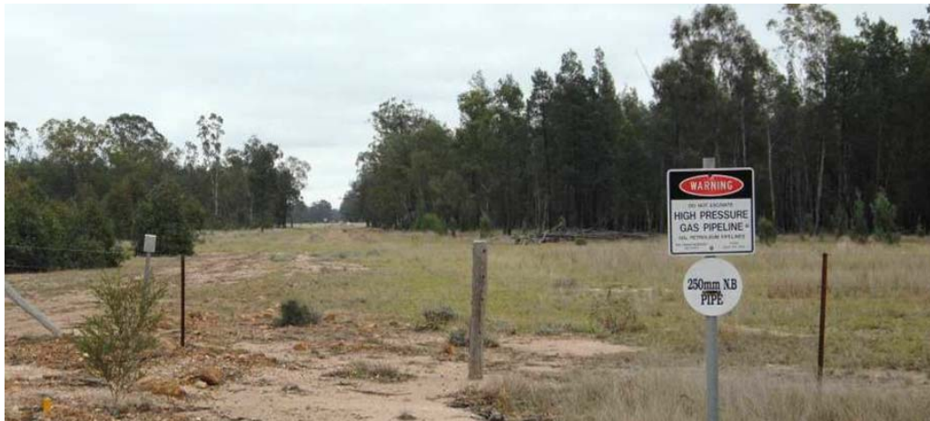
Figure 3.15.8 Roma to Brisbane Gas Pipeline – within less vegetated areas
