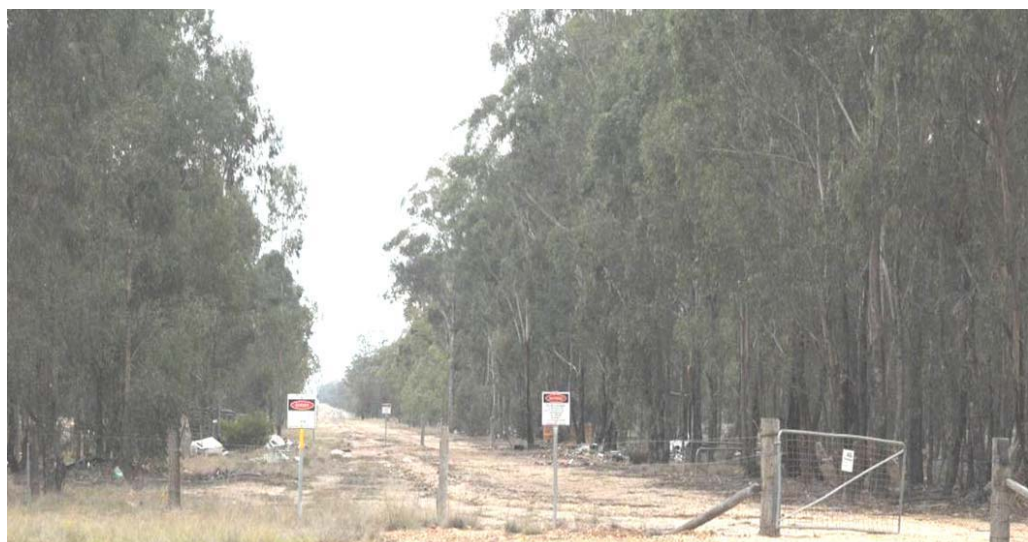
Figure 3.15.7 Roma to Brisbane gas pipeline – within a heavily vegetated area
