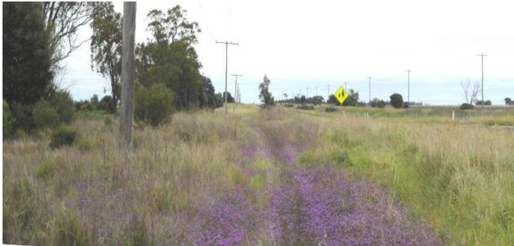
Figure 3.15.1 33 kV Power lines
