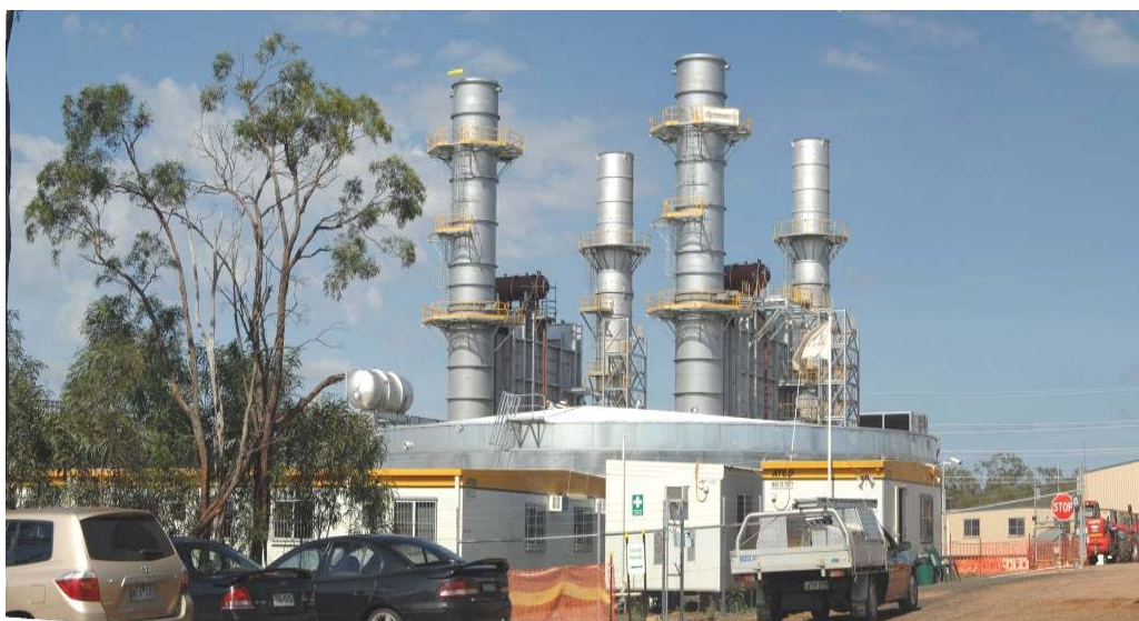
Figure 3.15.5 Condamine Power Station
