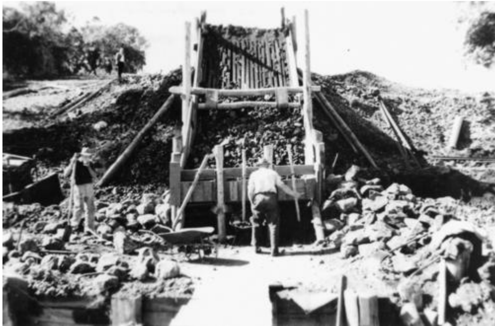
Figure 3.6 Road construction at Theodore c1930s (Banana Shire Council #ban 00096)
