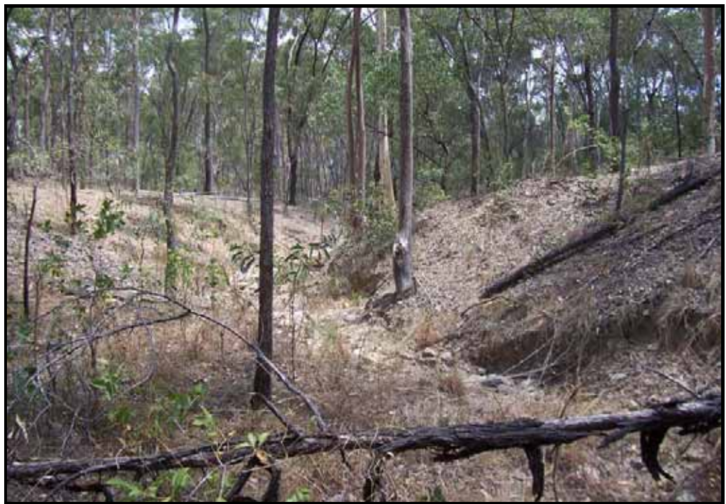
Photo 2 Evidence of erosion in the upper part of water course (flowing to the south)
