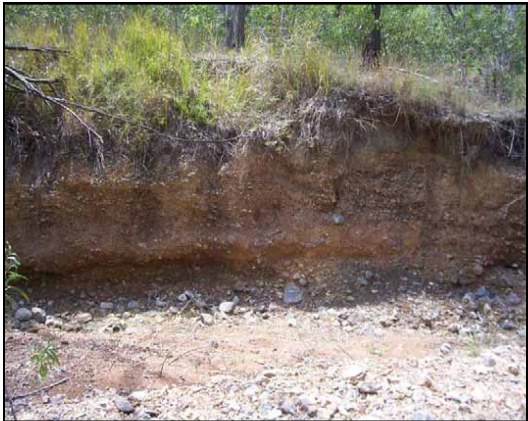
Photo 3 Erosion along creek bank, exposing overlying soil profile consisting of overbank alluvial deposits
