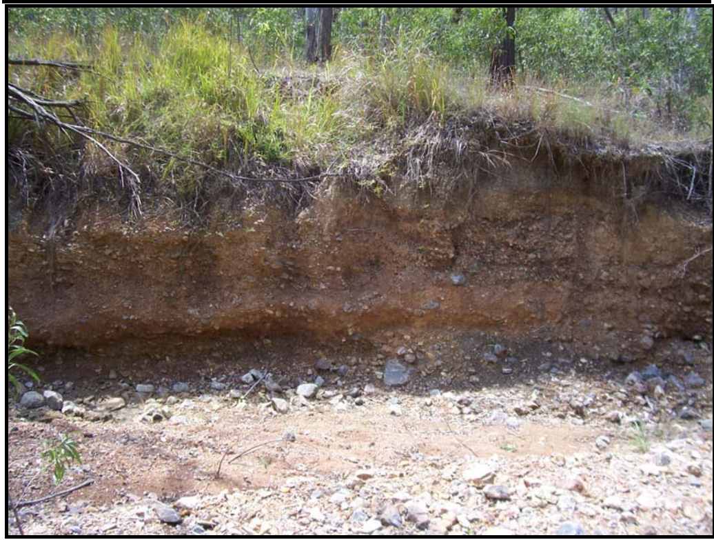
Plate 5.3.2 Erosion Along Creek Bank, Exposing Overlying Soil Profile Consisting of Overbank Alluvial Deposits
