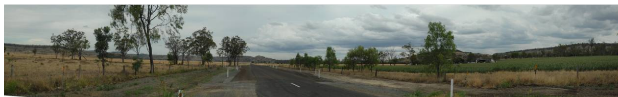
Figure 6.54 View looking east along the Burnett Highway
