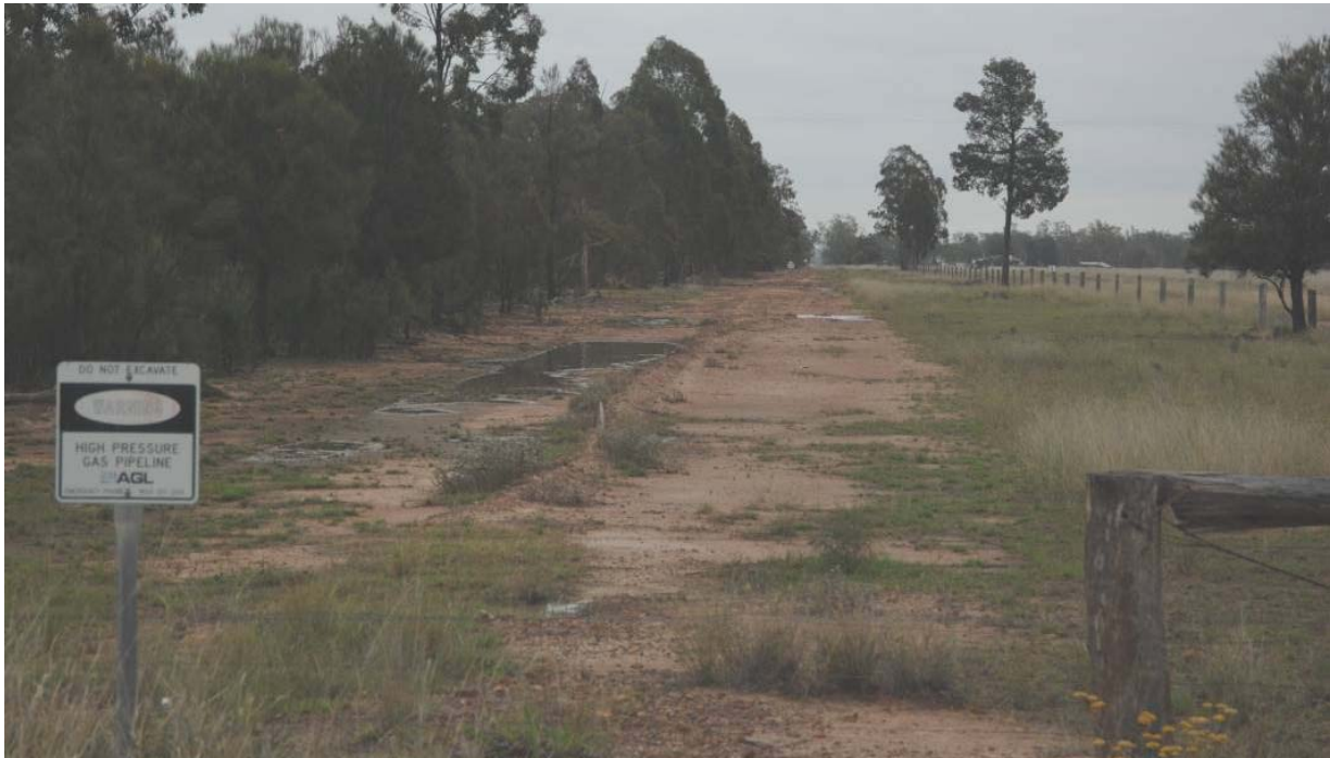
Figure 6.14 View looking west along existing Roma - Brisbane gas pipeline
