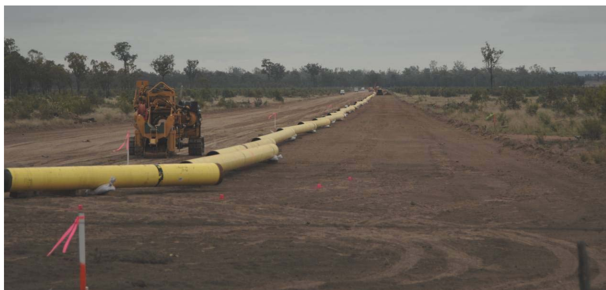
Figure 6.15 View looking north along the construction easement
