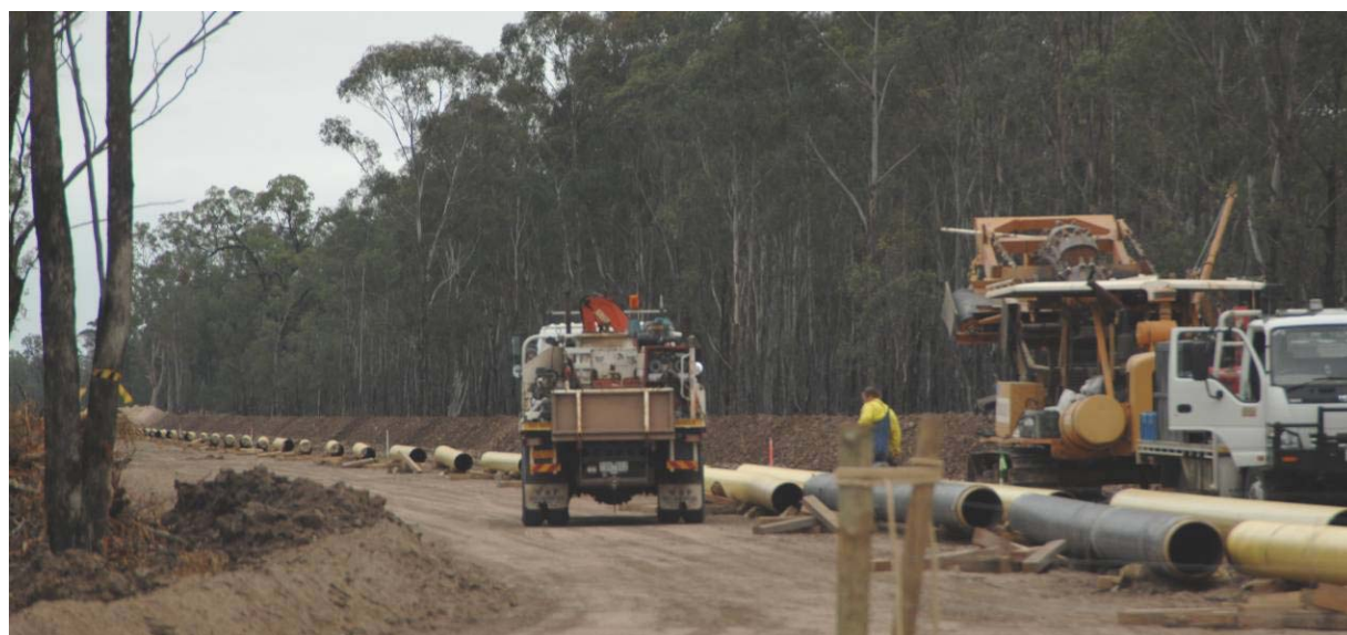
Figure 6.11 View looking east along an existing pipeline easement under construction
