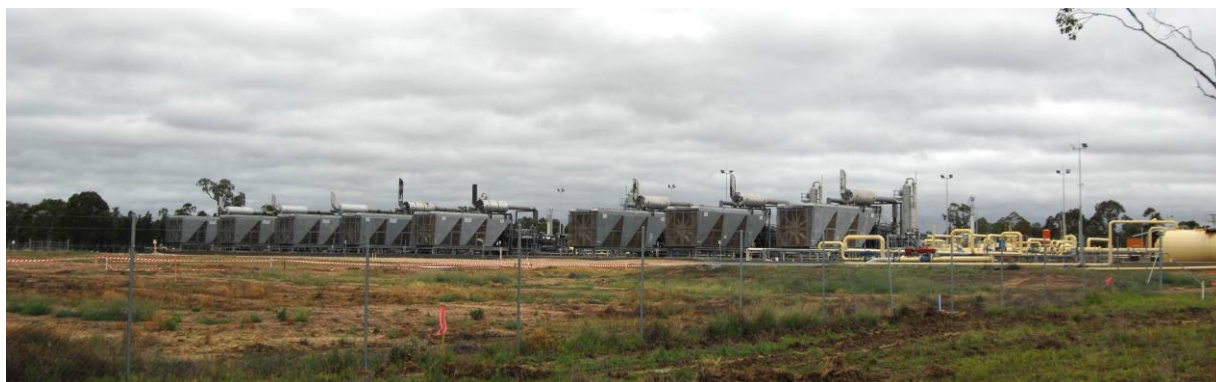
Figure 6.16 View looking west towards the existing gas compressor station.
