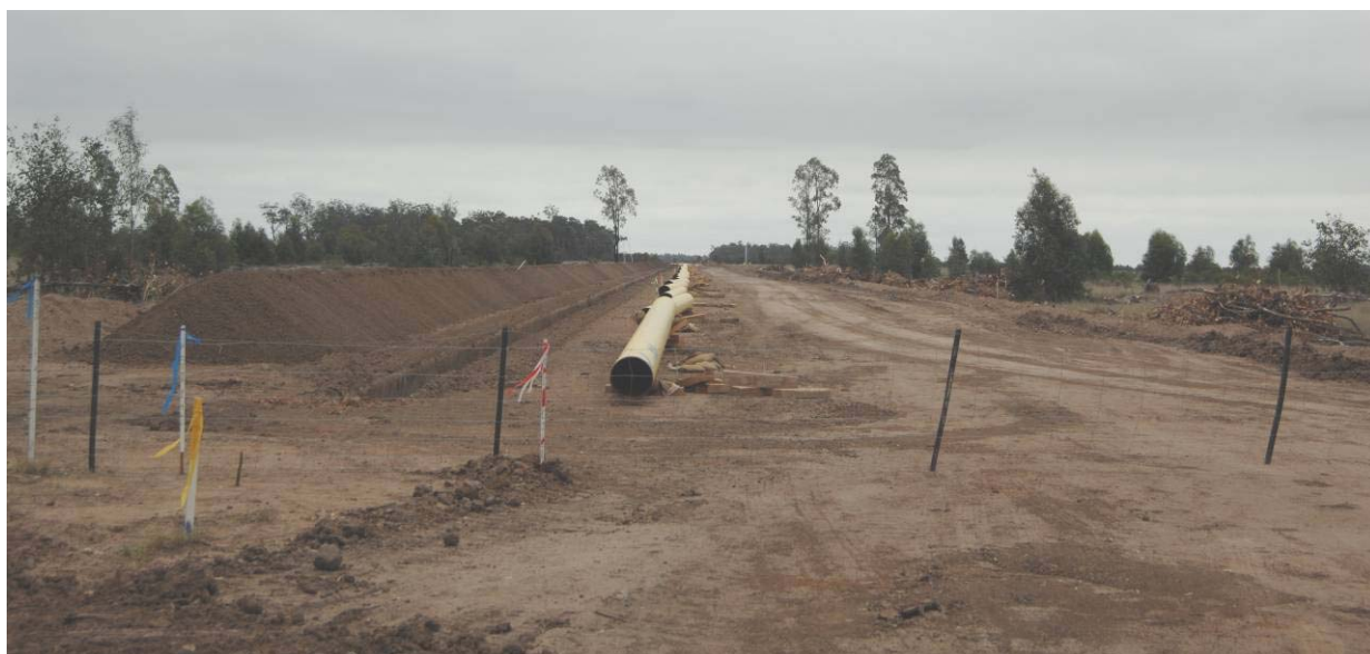
Figure 6.12 View looking west along pipeline easement under construction
