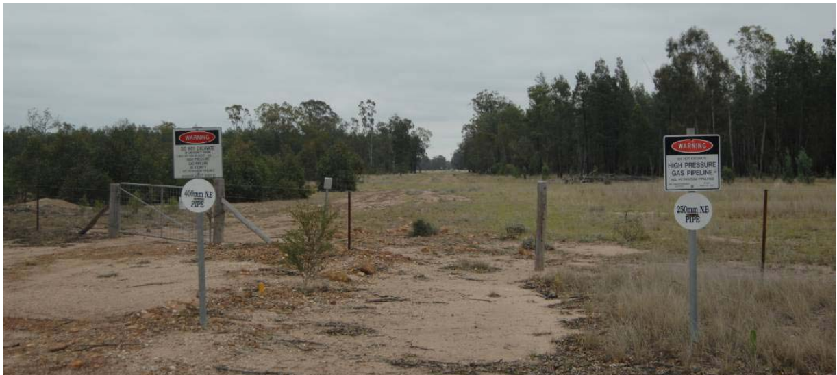
Figure 3.4 Roma to Brisbane Gas Pipeline corridor – cleared farmland
