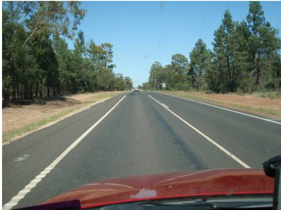
Figure 2.1 WARREGO HIGHWAY 18D (MILES–ROMA)—SEALED SHOULDERS
