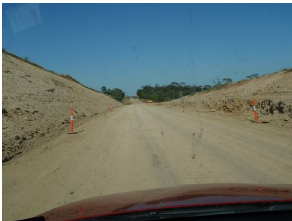
Figure 2.5 SECTION OF ROMA-TAROOM UPGRADE UNDER CONSTRUCTION
