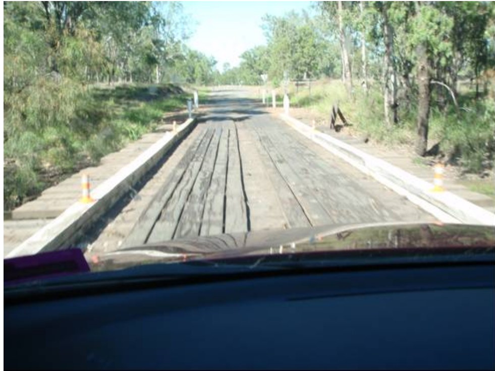
Figure 2.6 A ONE-LANE TIMBER BRIDGE ON THE ROMA–TAROOM ROAD
