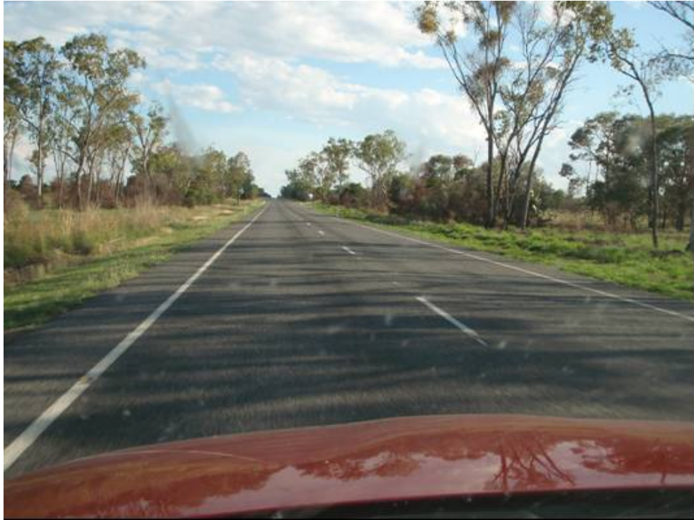
Figure 2.2 LEICHHARDT HIGHWAY 26B (TAROOM-MILES)—SEALED SHOULDERS
