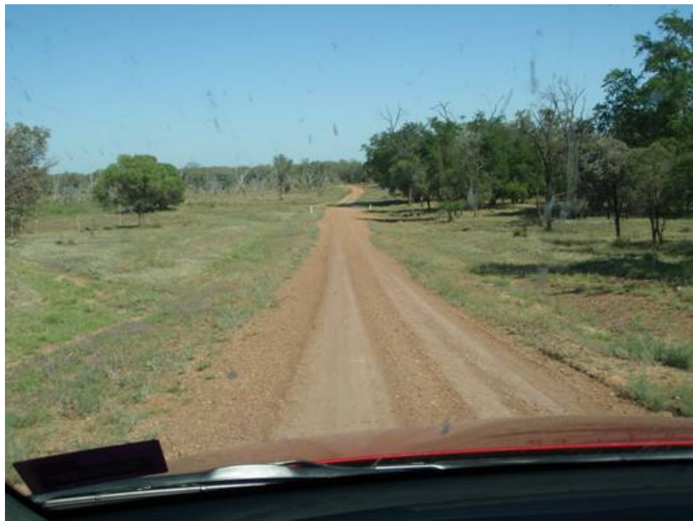
Figure 2.7 INJUNE-ROMA CONNECTION ROAD—PAVED AND UNSEALED
