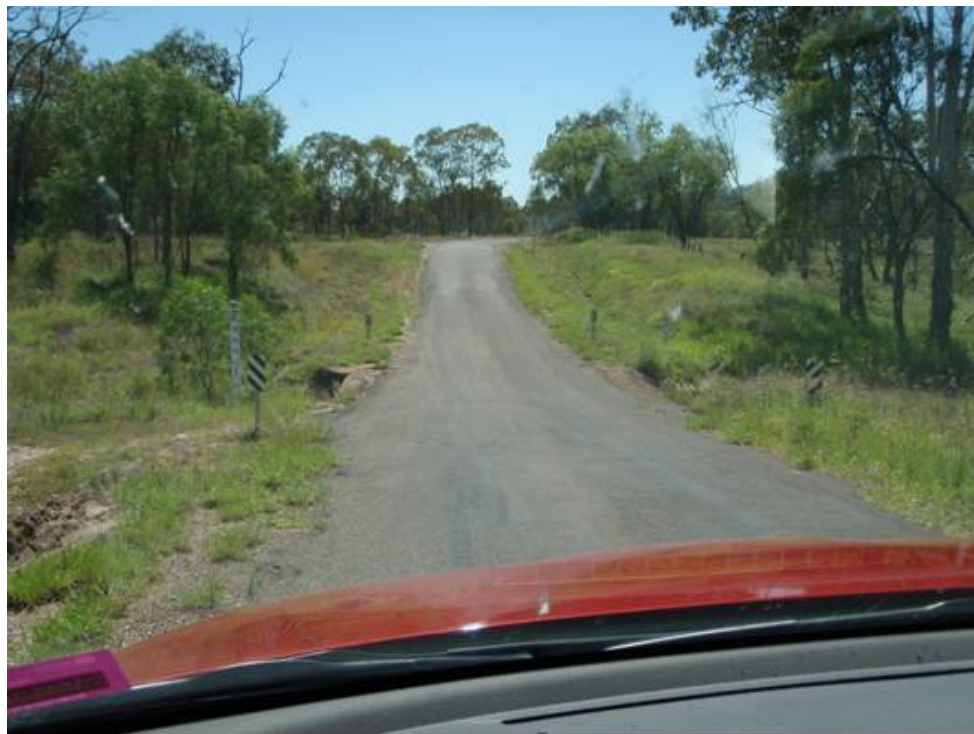
Figure 2.4 JACKSON-WANDOAN ROAD—SINGLE LANE BITUMEN FLOODWAY
