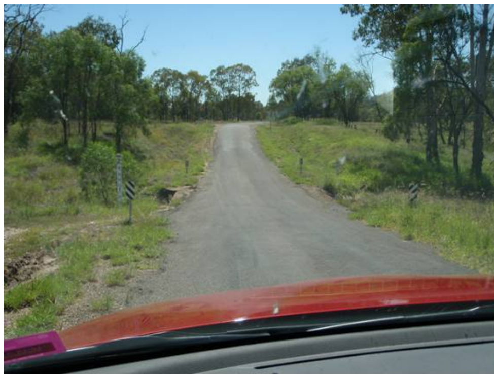
Figure 2.5 JACKSON-WANDOAN ROAD—SINGLE LANE BITUMEN FLOODWAY
