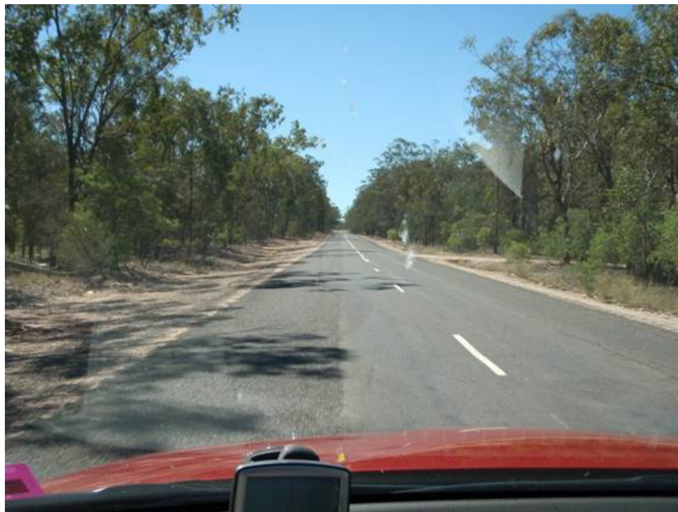
Figure 2.4 KOGAN-CONDAMINE ROAD—UNSEALED SHOULDERS
