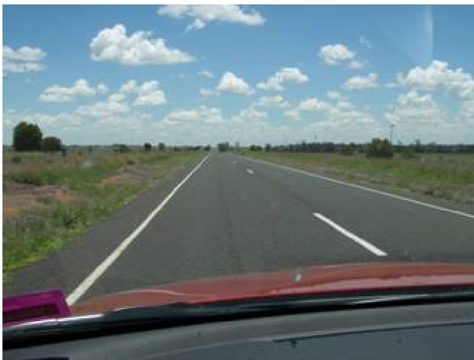
Figure 2.3 LEICHHARDT HIGHWAY 26B (TAROOM—MILES)—SEALED SHOULDER
