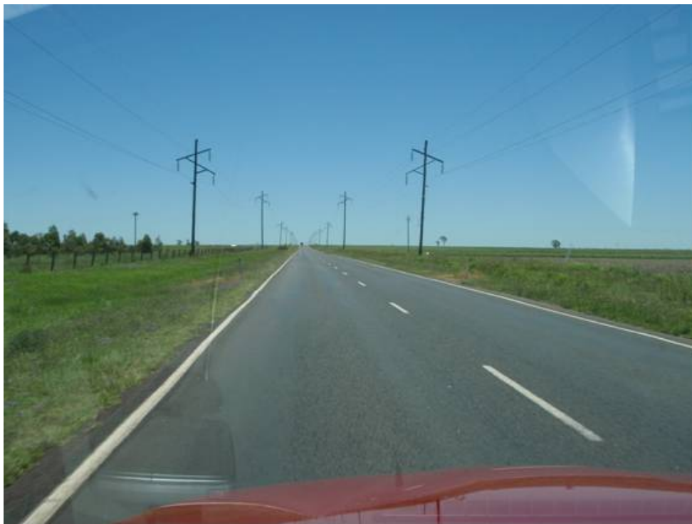
Figure 2.2 WARREGO HIGHWAY EAST OF DALBY—UNSEALED SHOULDERS
