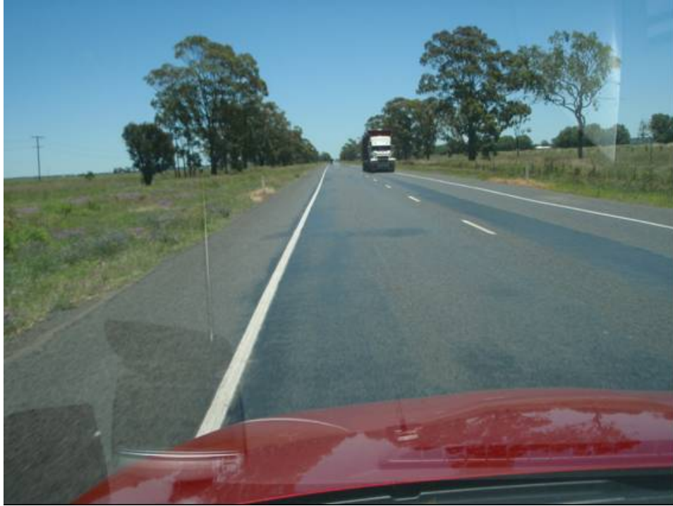
Figure 2.1 WARREGO HIGHWAY WEST OF OAKEY—2 M WIDE SEALED SHOULDERS
