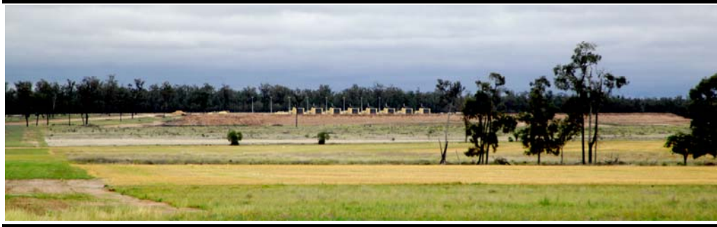
Plate 3.15.2 Compressor Station at 750 m
