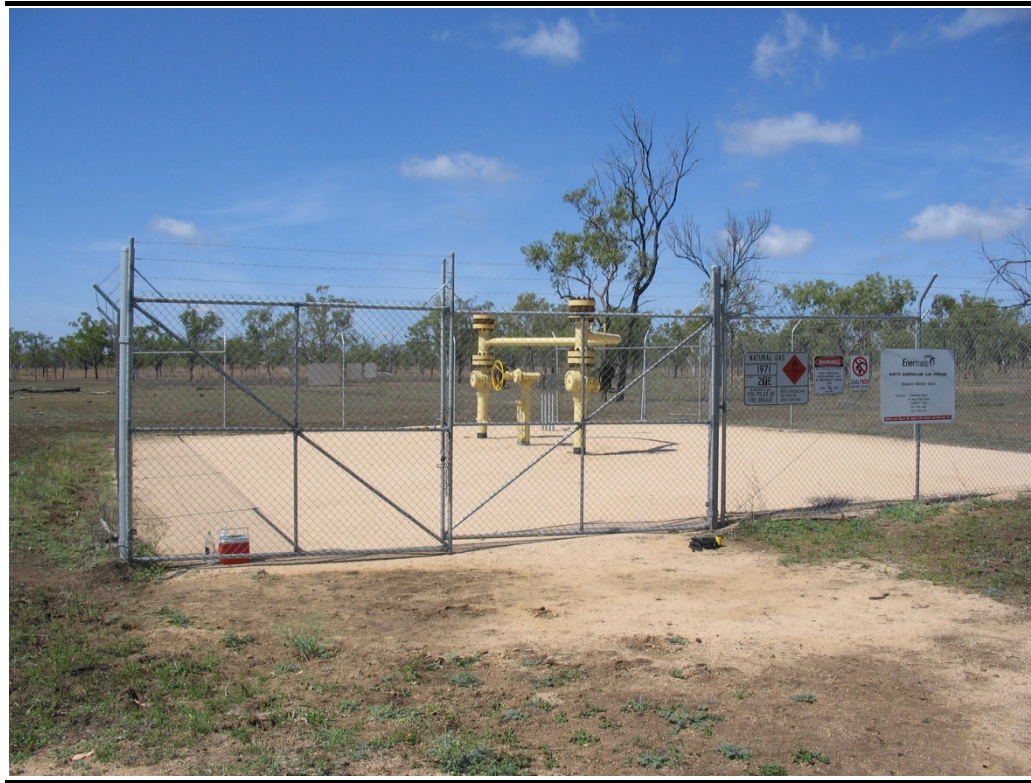
Plate 2.12.3 Typical Scraper Station
