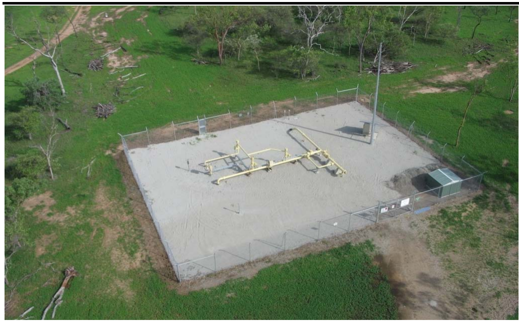
Plate 2.12.3 Typical Scraper Station
