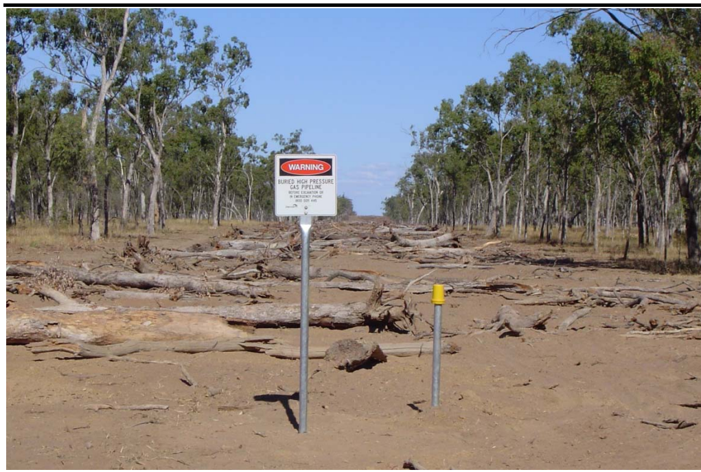
Plate 2.12.1 Typical CP Test Point and Marker Post
