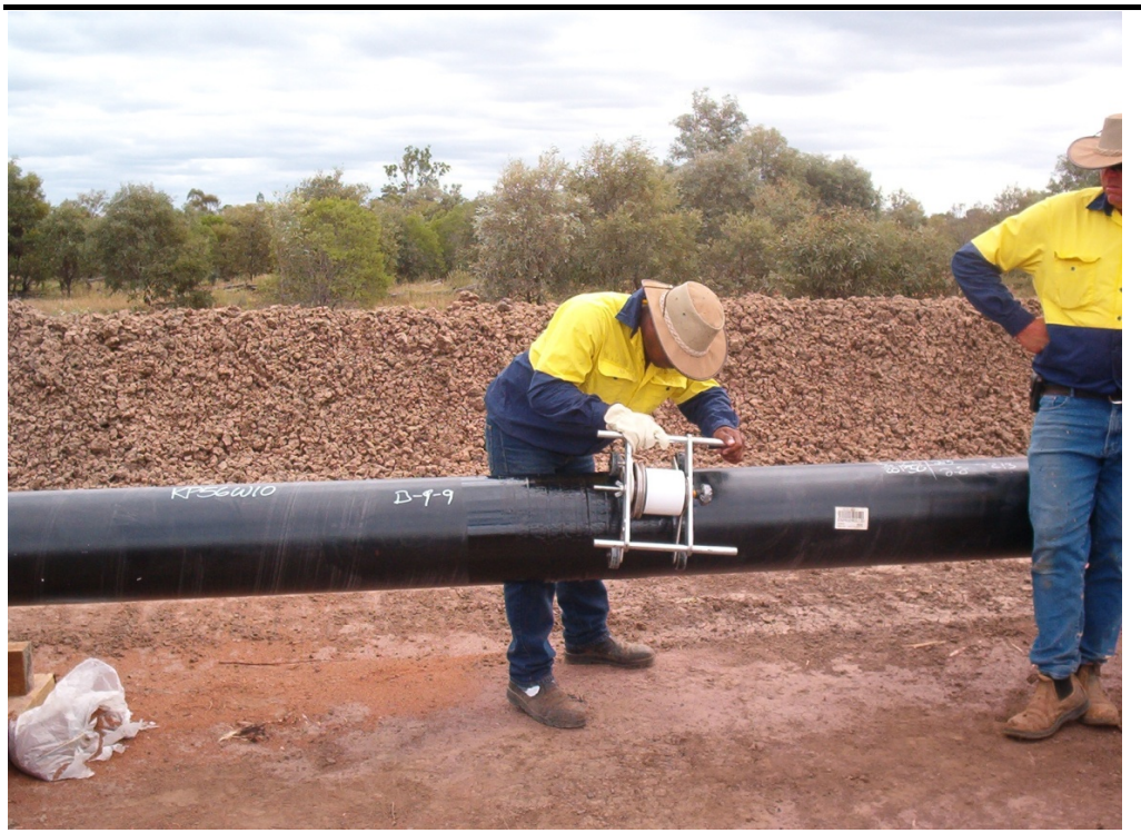
Plate 2.12.8 Field Coating Join
