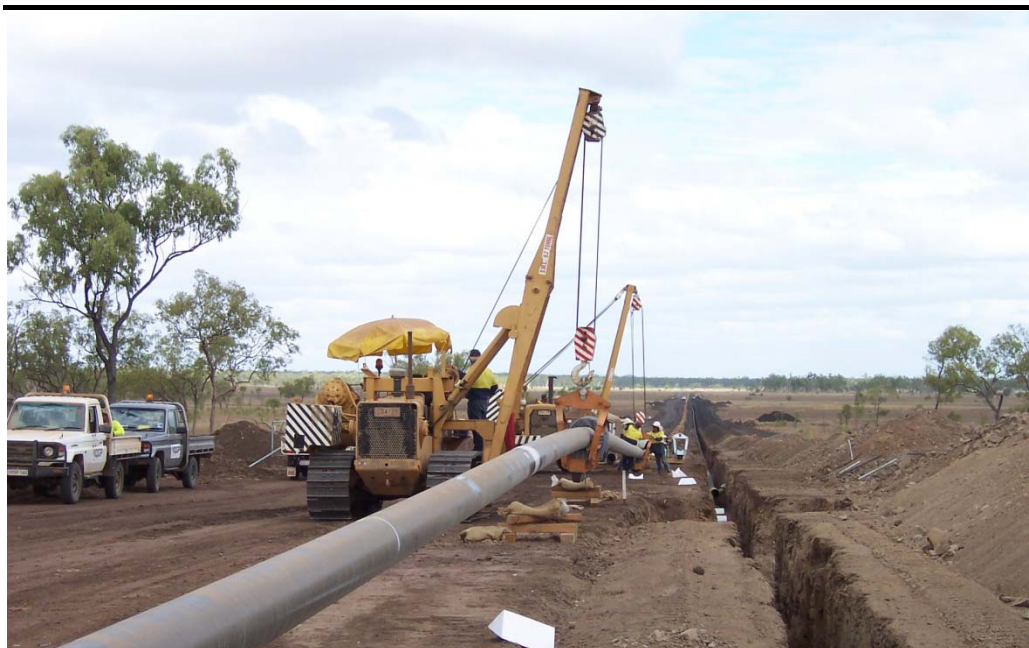
Plate 2.12.9 Pipe Being Lifted into Place
