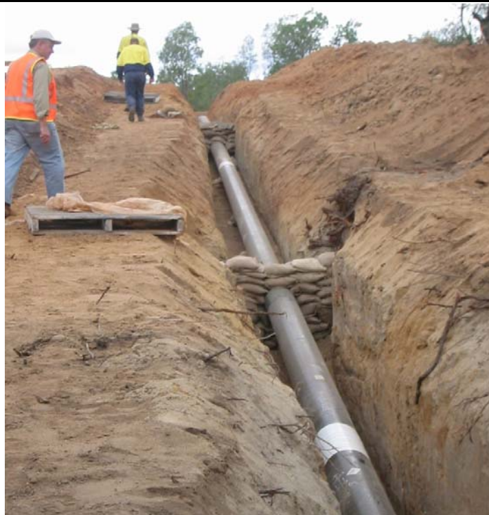
Plate 2.12.10 Typical Trench Breaker 1
