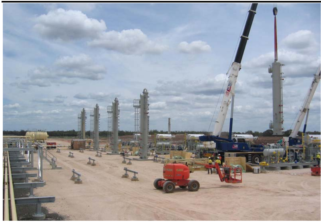
Plate 2.11.4 Installation of TEG unit at CPP
