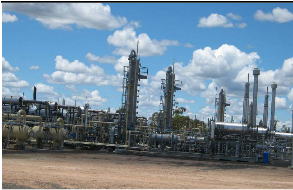
Plate 2.7.7 CPP showing TEG units in the Foreground
