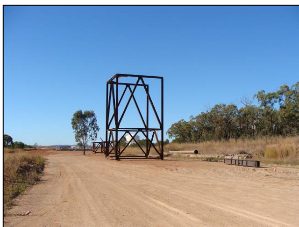
Figure 6: HI-1 Hardstand area / roadway
