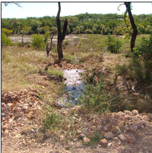
Figure 8: HI-3 Overflow channel
