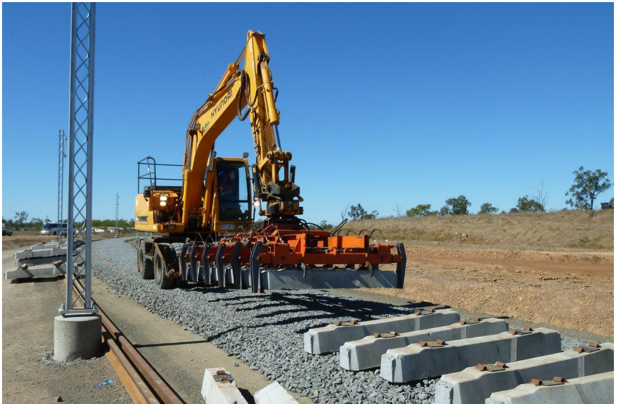
Figure 2-9 Excavator with octopus attachment
