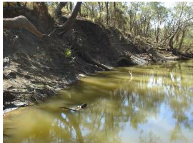
f) IZ6 – Dawson River. Erosion of terraces
