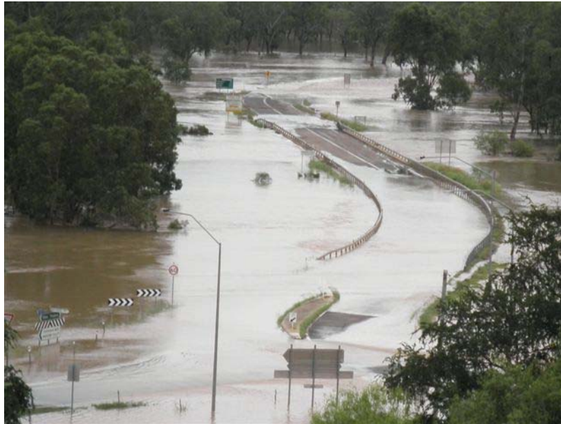
Figure 14-40 Flooding at the Leichardt Highway Bridge at Taroom (March, 2010)
