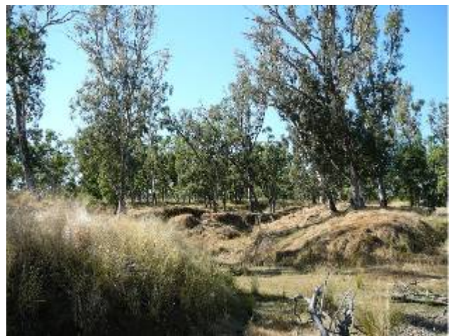
b) Streambank erosion in Bungaban Creek downstream of the Nathan Road crossing
