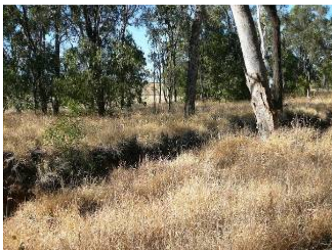
a) Eroded drain in the road reserve adjacent to Nathan Road
