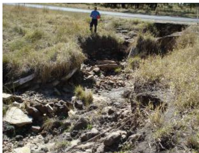
b) Erosion downstream of culvert
