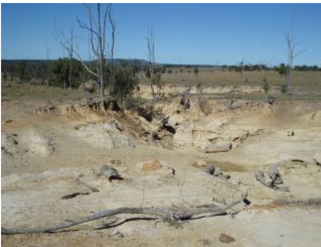
a) Gully erosion
