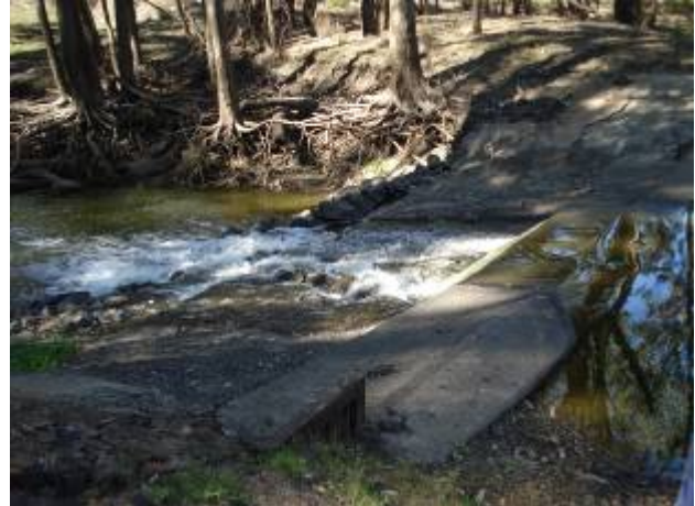
b) IZ5 – Dawson River, Small weir downstream of Glebe Weir that channels flow into anabranch.
