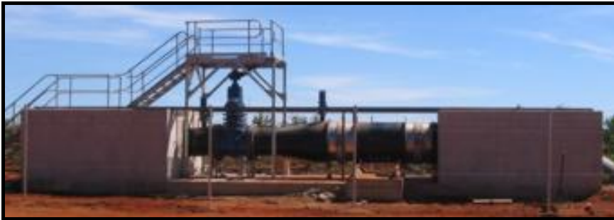
Figure 2-24 Typical swab insertion and removal station
