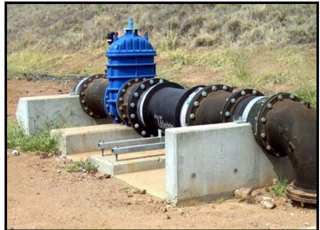
Figure 2-21 Control valve
