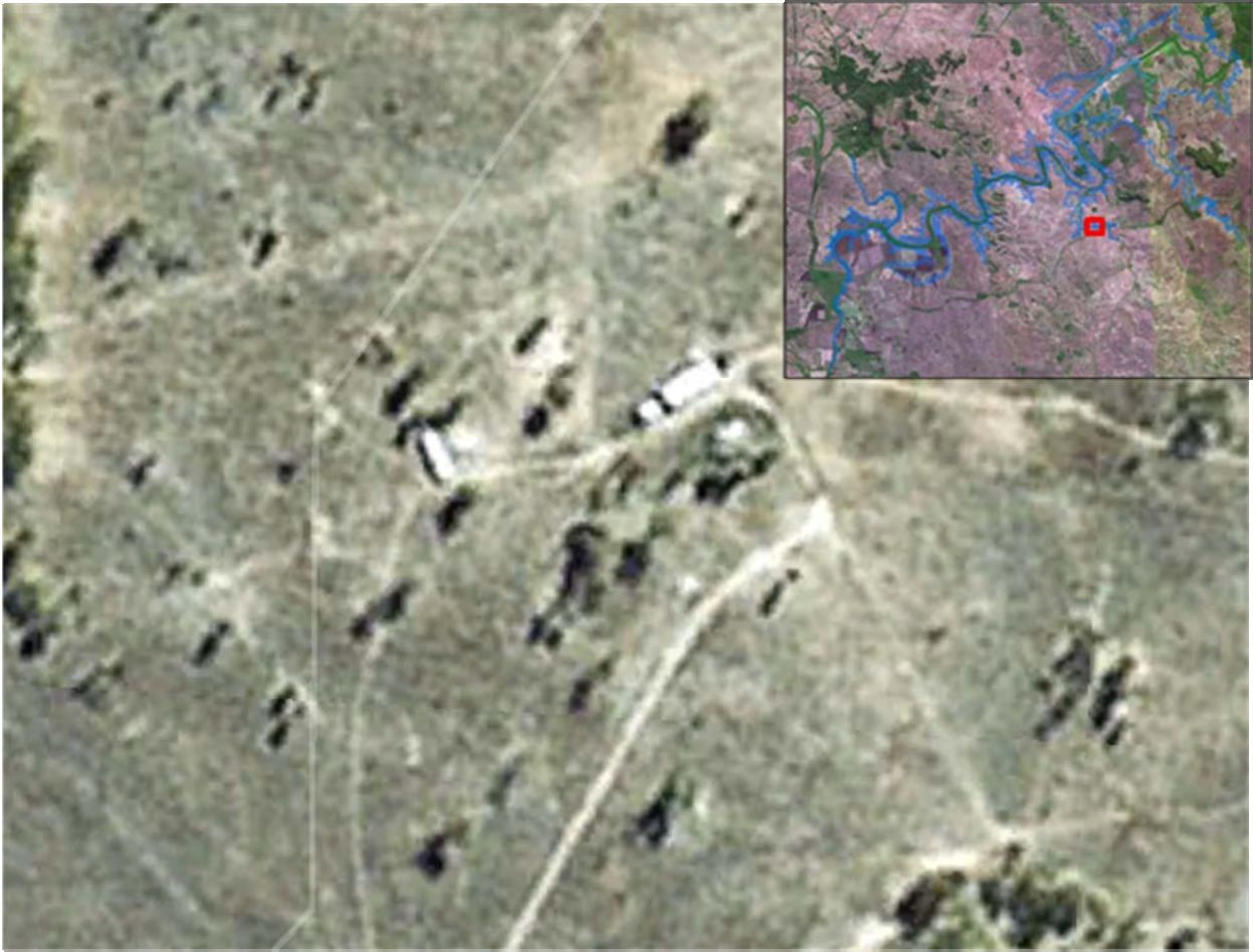
Figure 8A-16 Buildings 2 (Google Earth Pro 2010)
