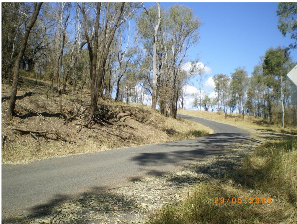
Figure 16-6 A typical bitumen sealed local road in the study area
