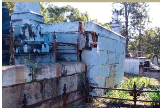
Figure 19: Badly cracked monumental masonry in Toowong Cemetery
