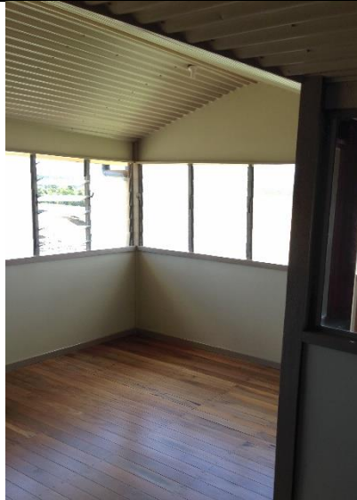
Figure 37: Original enclosed veranda with louvered windows, northern and western elevations. Thorp, 2017.
