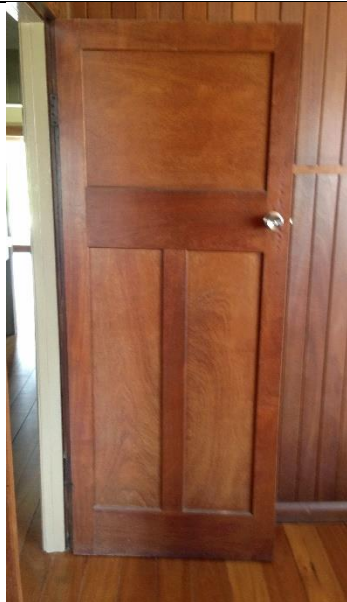
Figure 38: Main bedroom: original wall cladding, silky oak doors and mixed rainforest timber floor boards. Thorp, 2017.
