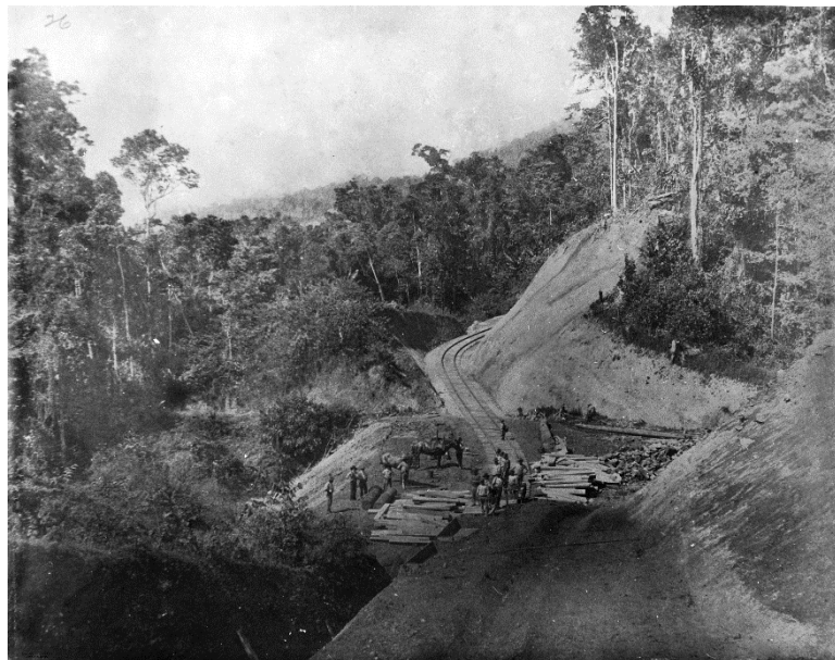
Figure 6: Workers laying sleepers and lines during construction of Cairns to Myola railway, c. 1890. JOL: 22620.
