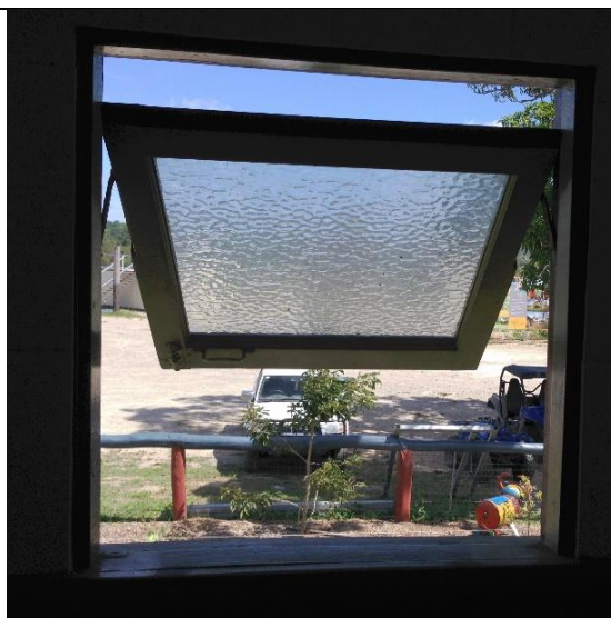
Figure 35: Original hopper window, stove alcove: southern elevation. Thorp, 2017.
