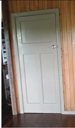
Figure 36: Original opening between lounge and enclosed veranda. Now a cupboard. Thorp, 2017.
