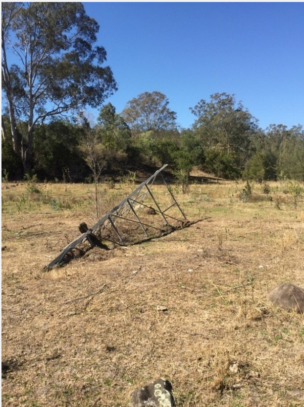
Photograph 6.30 G2H-19-H24 broken metal windmill tower
