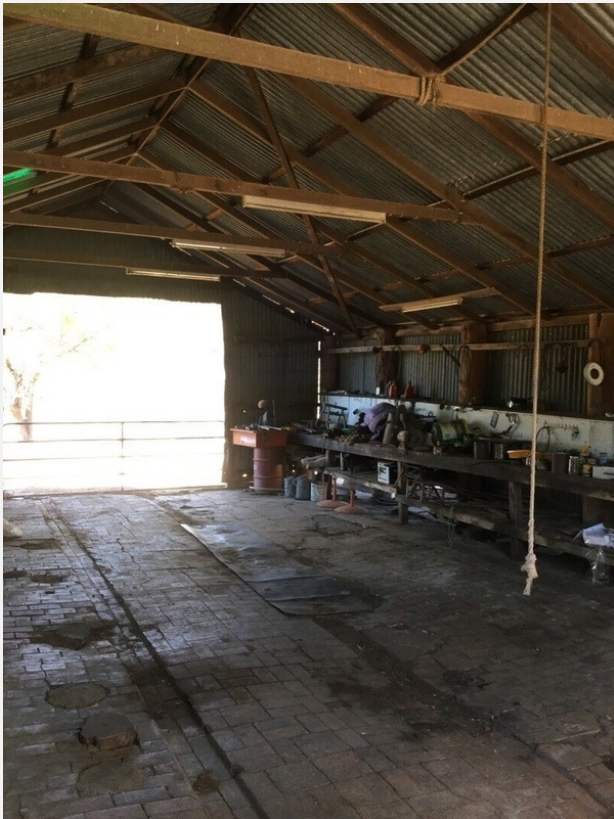
Photograph 6.37 G2H-19-H26 shed 1 original brick floor and timber stumps visible
