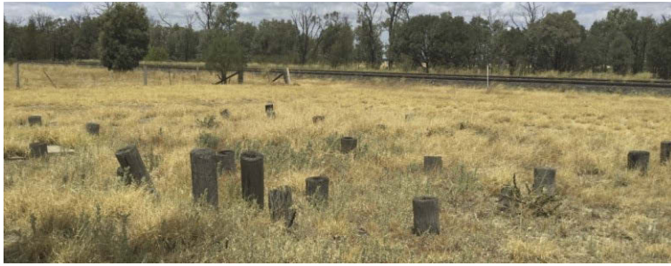
Photograph 6.1 Building stumps (B2G-19-H01)
