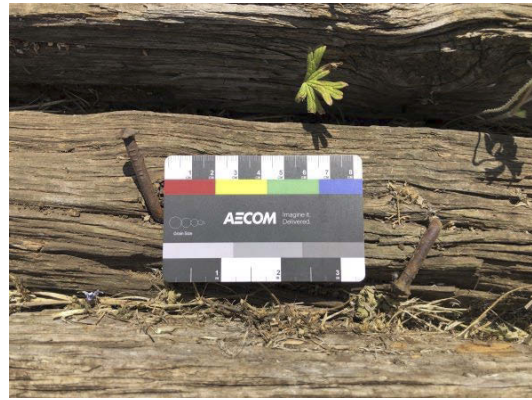
Photograph 6.47 Roseheaded wire nails in fence remnants (B2G-21-H13)
