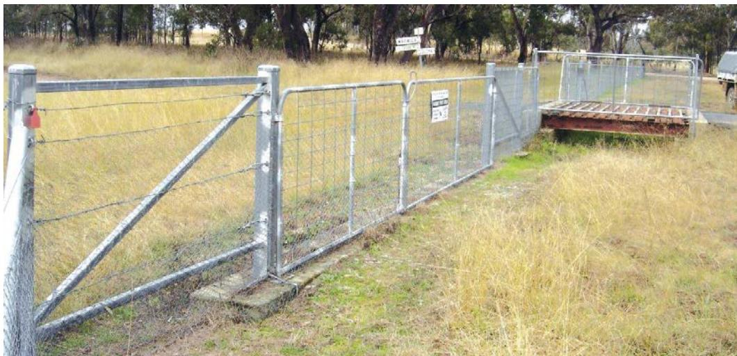
**Photograph 3.1 Example of a rabbit-proof fence design with a gate trap**
