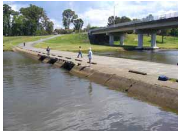
Plate 10:5: Barrier Downstream of Hinze Dam
