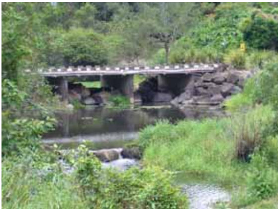
Plate 10:4: Barrier Downstream of Hinze Dam
