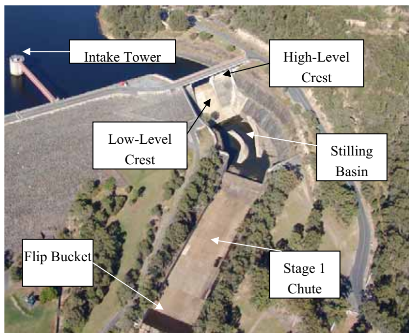
Plate 10:8: Stage 2 Spillway Arrangement and Structure Locations
