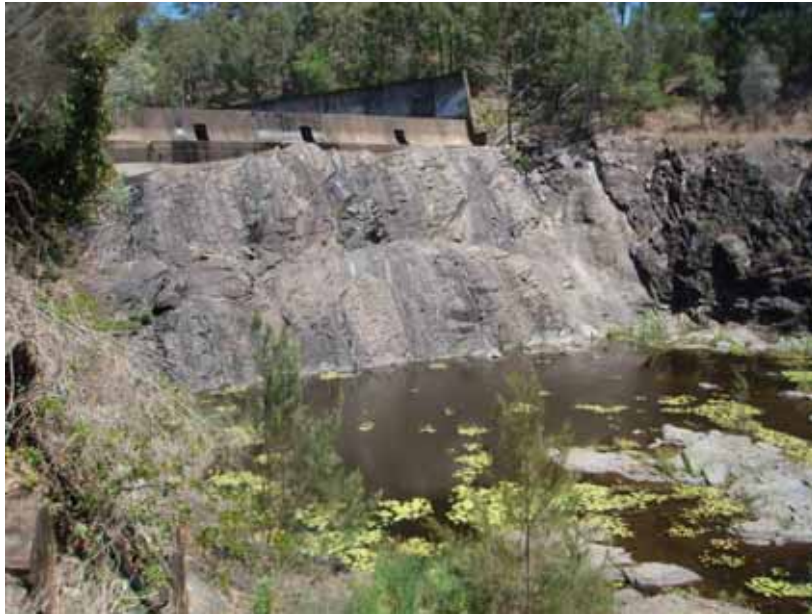
Plate 10:10: Existing Plunge Pool Below the Downstream Spillway Chute
