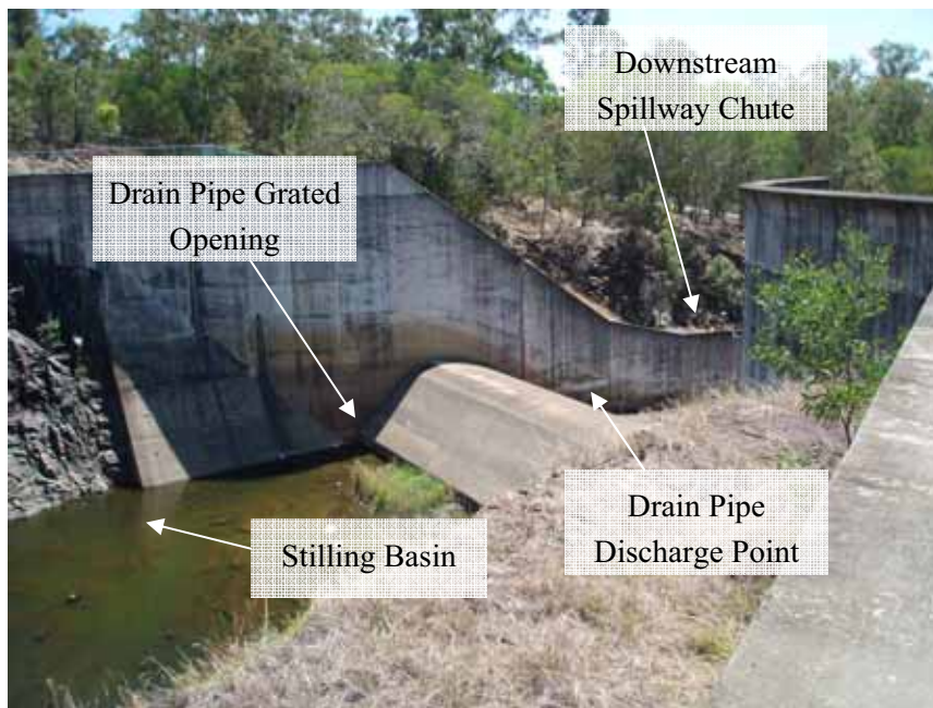
Plate 10:9: Existing Drainage Arrangement for the Stilling Basin
