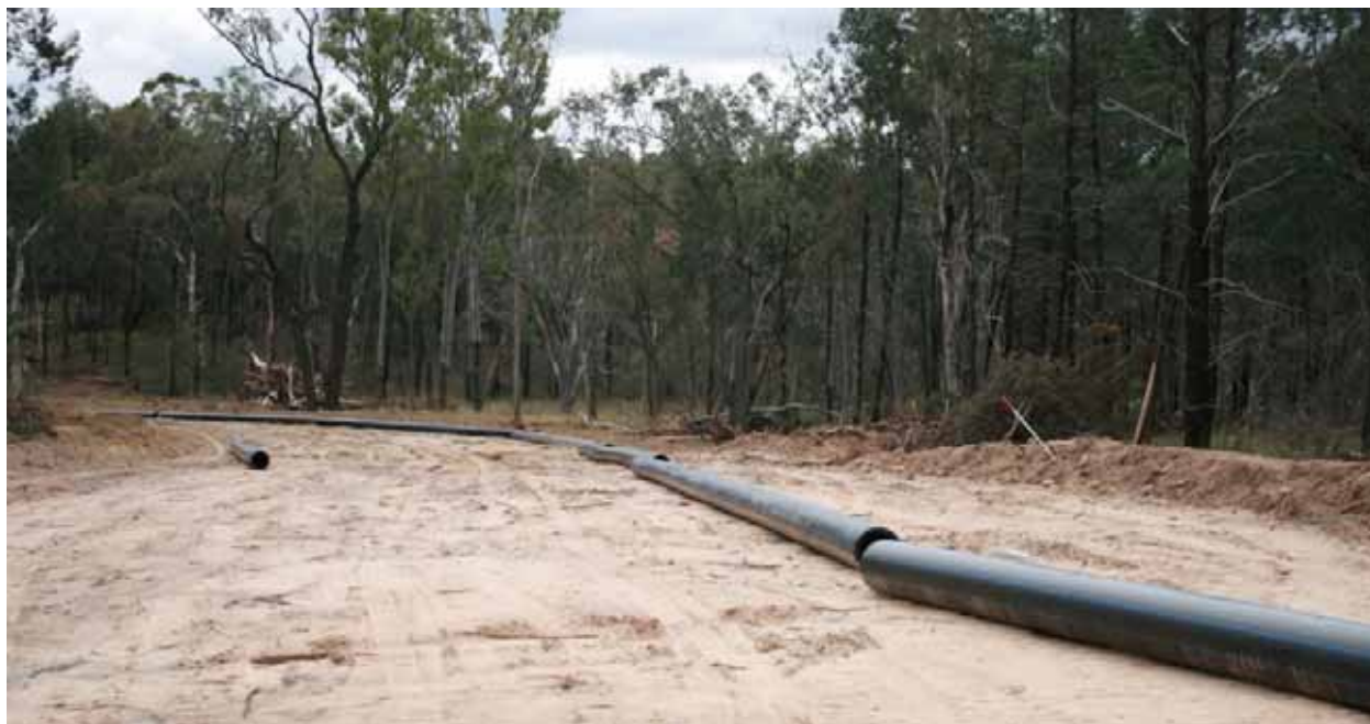
Plate 25 Gas collection pipeline laid out along easement in forest area prior to trenching and installation
