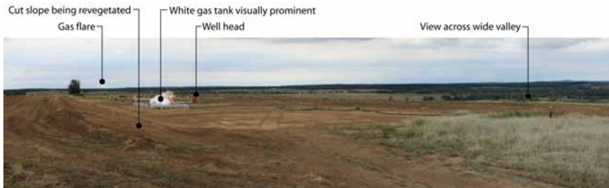
Plate 22 Production well on ridge top with cut and fill slopes prior to revegetation
