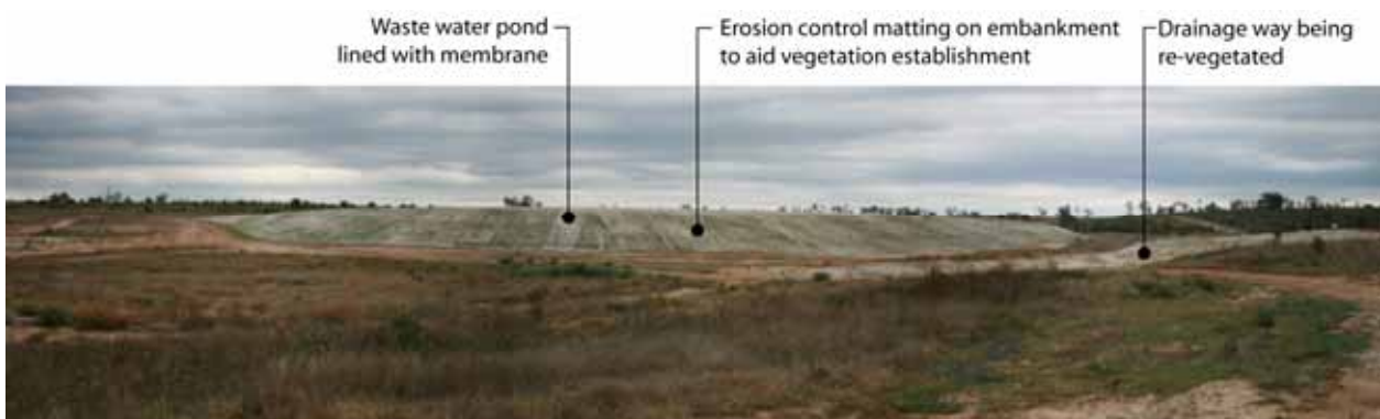
Plate 31 Water storage dam embankment with erosion control matting used to establish a protective grass cover
