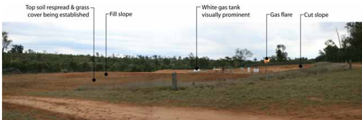
Plate 20 Production well site on undulating landform showing cut and fill slopes prior to revegetation
