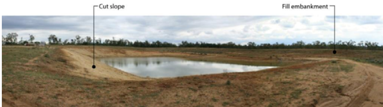
Plate 29 Water storage dam constructed near Coxon Creek
