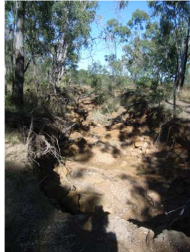
Photo: Downstream Channel
