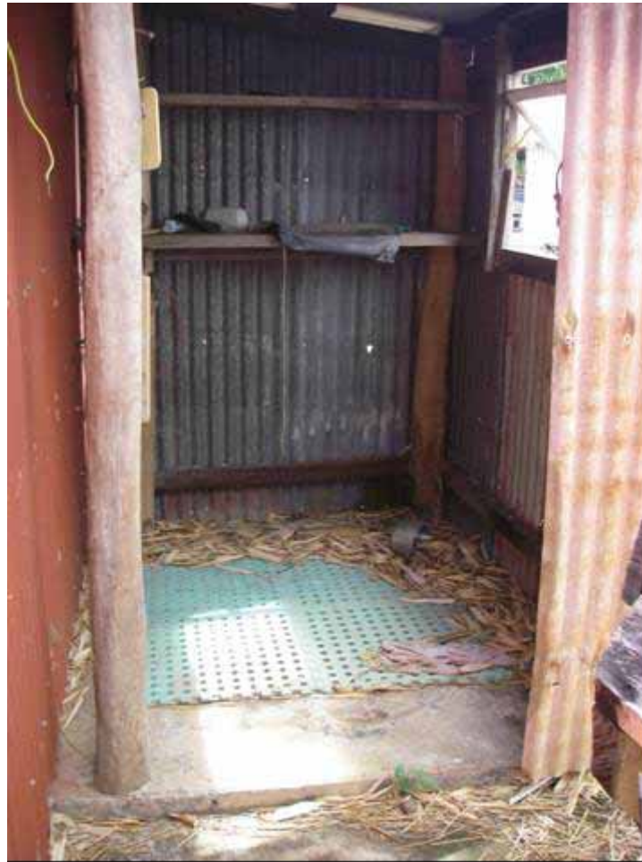
Plate 3-8 Generator shed at Fisherman's Hut
