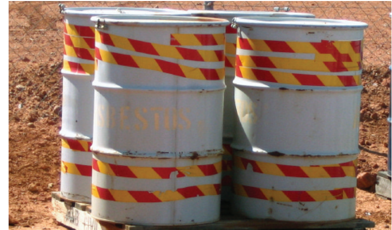
Asbestos in drums awaiting disposal.
