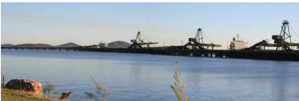
Plate 8.12.5 LCZ 5 - Coal Loading Port Facilities
