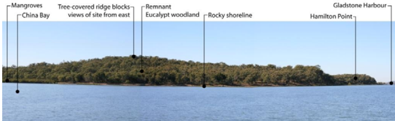
Plate 8.12.12 View to North-eastern Portion of the LNG Facility Site from China Bay
