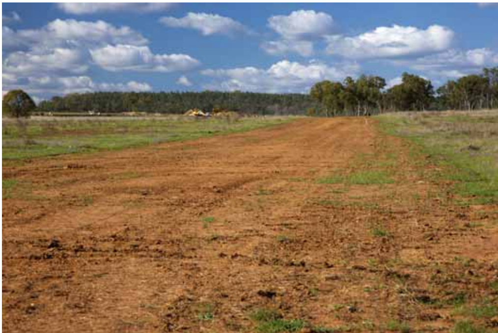
Plate 7.12.2 Typical pipeline easement after backfilling trench and prior to revegetation works
