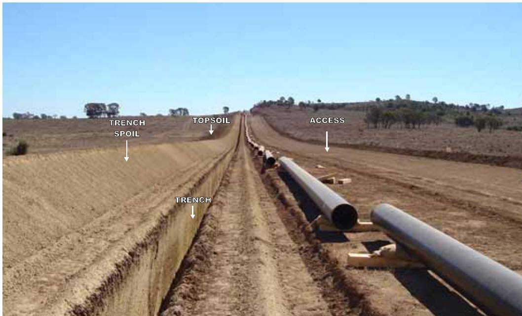
Plate 7.12.1 Typical trench with 'pipe string' laid out ready for installation
