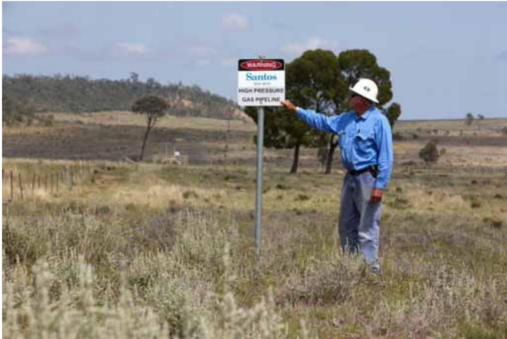
Plate 7.12.3 Rehabilitated pipeline easement showing pipeline marker and mainline valve
