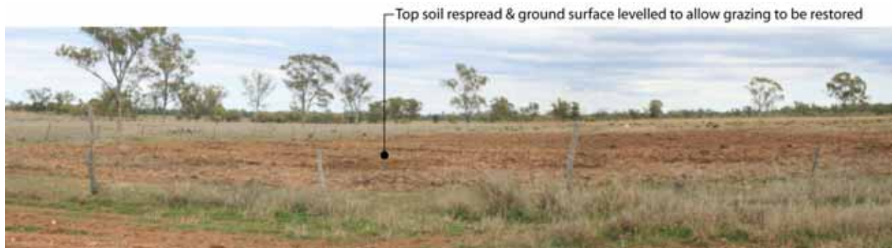
Plate 6.12.37 Exploration Drilling Site in Grazing Paddock after Regrading and Top Soiling
