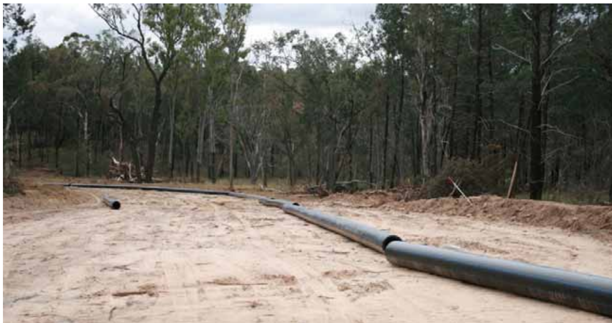
Plate 6.12.25 Gas Collection Pipeline Laid Out Along Easement in Forest Area Prior to Trenching and Installation
