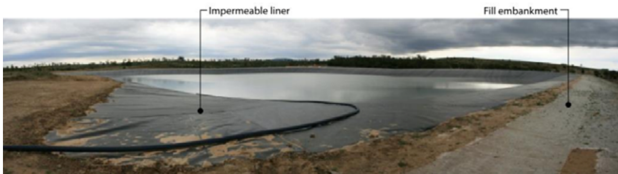
Plate 6.12.29 Water Management Pond Constructed with Impermeable Liner
