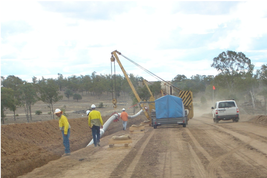
Figure 3.7.3 Lowering-in of Pipeline
