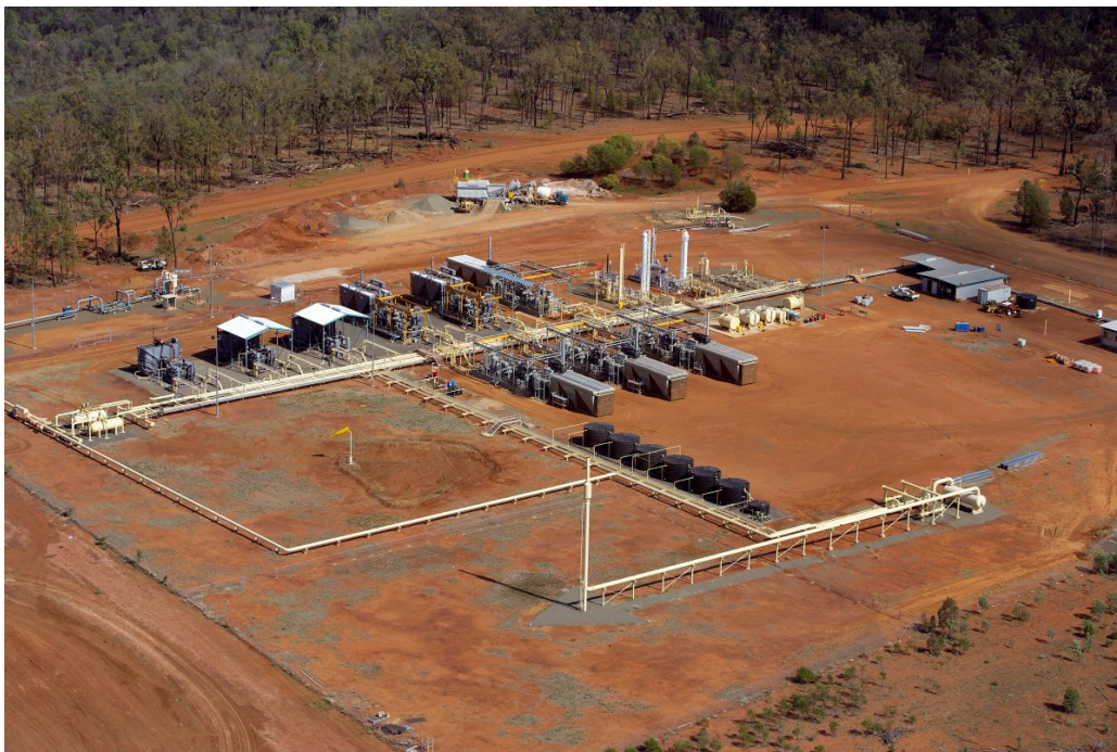
Figure 3.6.11 Centralised Compression and Water Treatment Facility - Fairview
