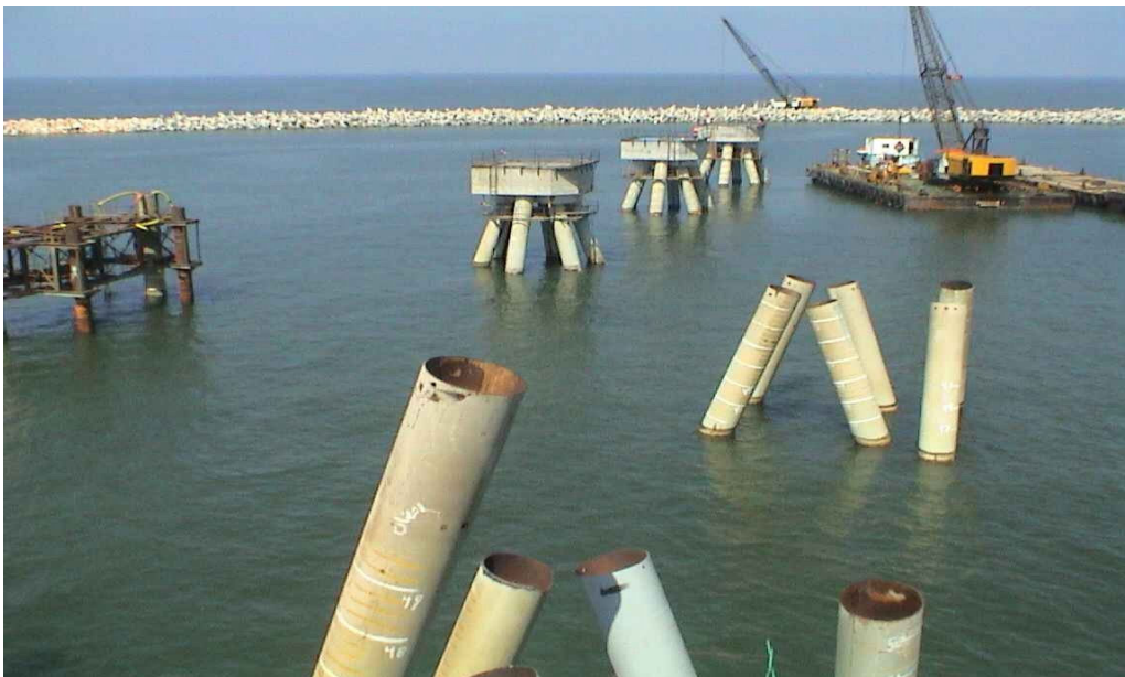
Figure 3.8.3 Floating Crane Barge Placing Pile Caps for Mooring Dolphins
