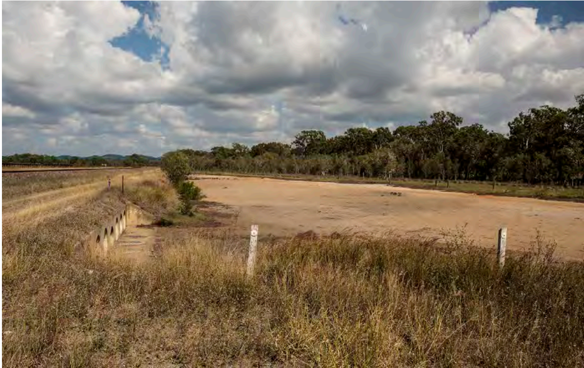
Figure 5-5: Project site drains to a natural basin before it overflows through the culverts
