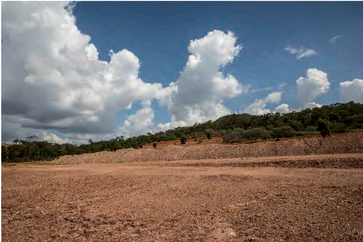
Figure 5-3: Erosion gullies in red fine gravel site surface
