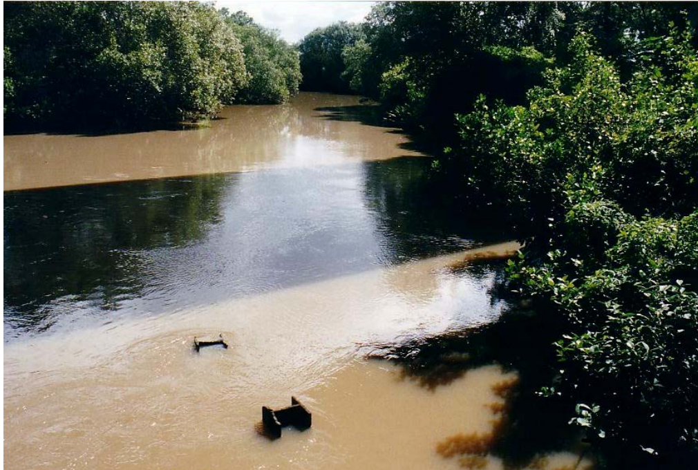
Figure 8 : Remnant metal ‘I-beam’ girders in Bulimba Creek.
