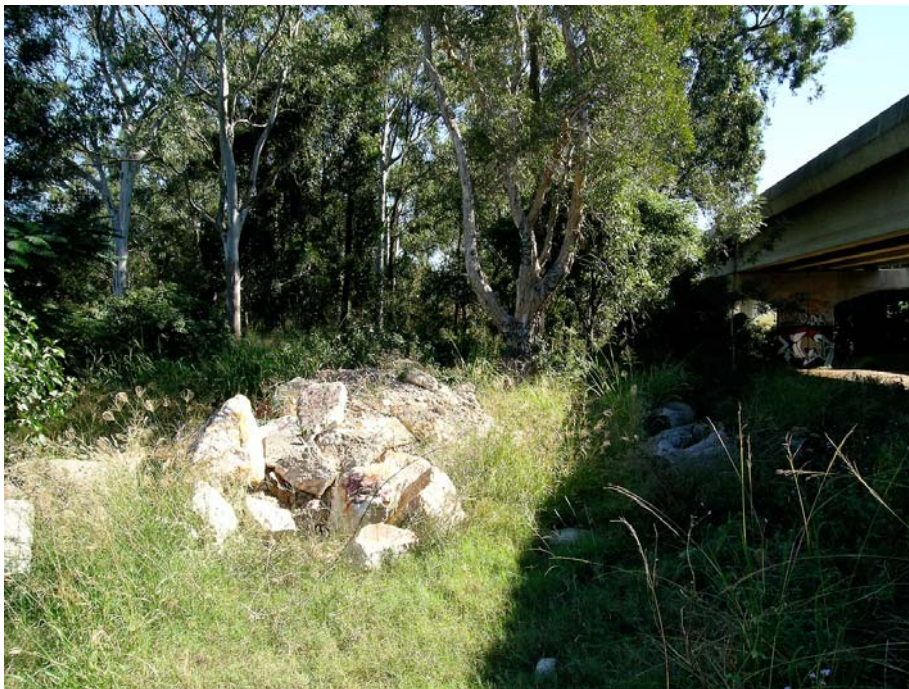
Figure 7: Examples of imported refuse in front of a stand of remnant eucalypts beside the Gateway Motorway on the south bank of Bulimba Creek
